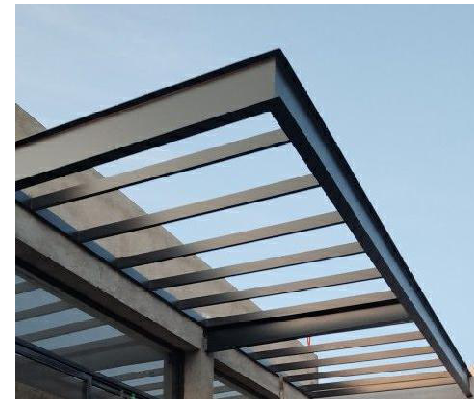
BLACK PAINTED STEEL CANOPY W/ LAMINATED GLAZING
