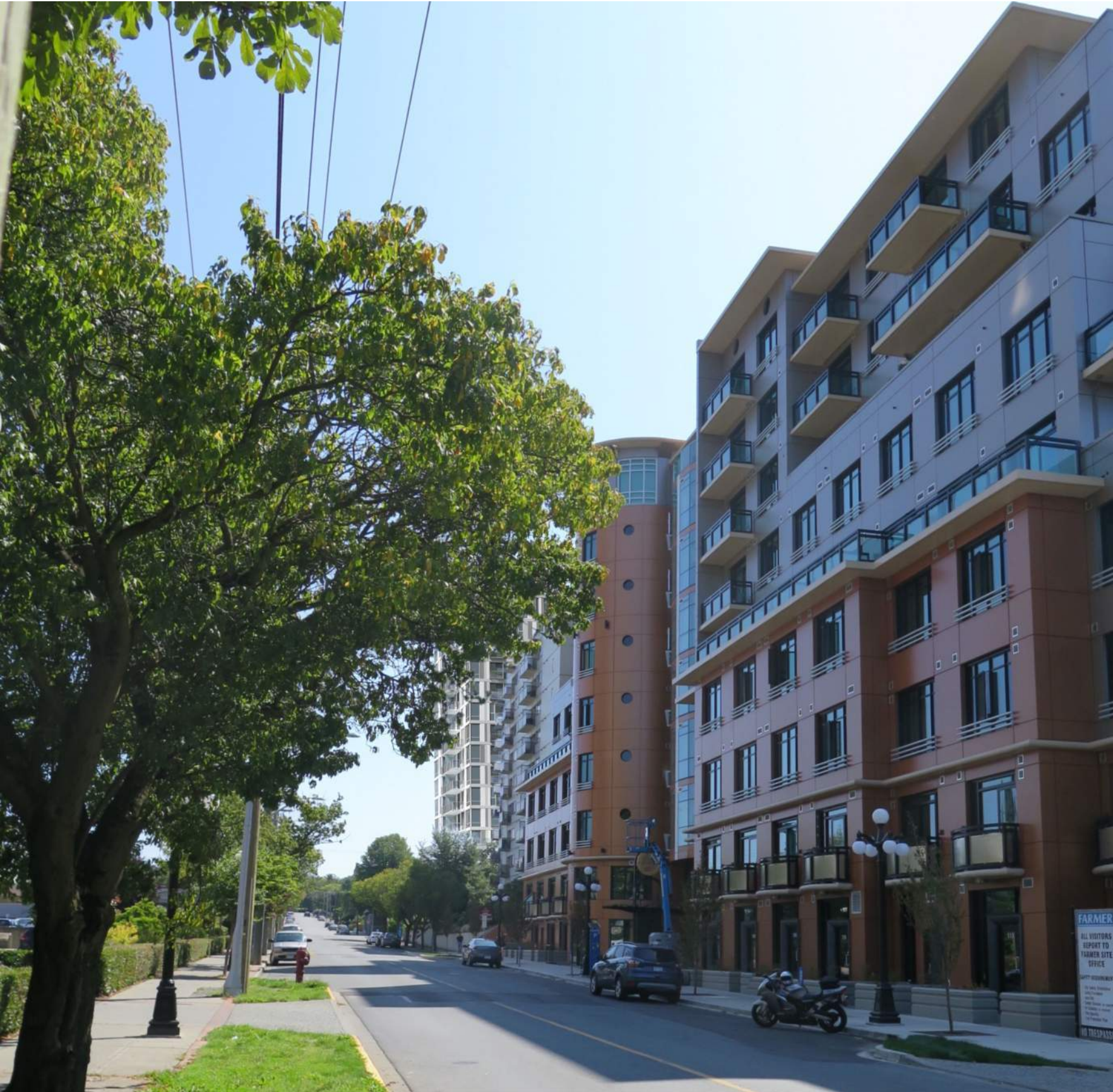
B View Street Looking East
