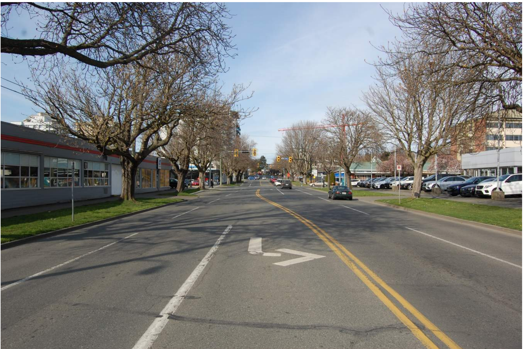
1. Cook Street Looking South
