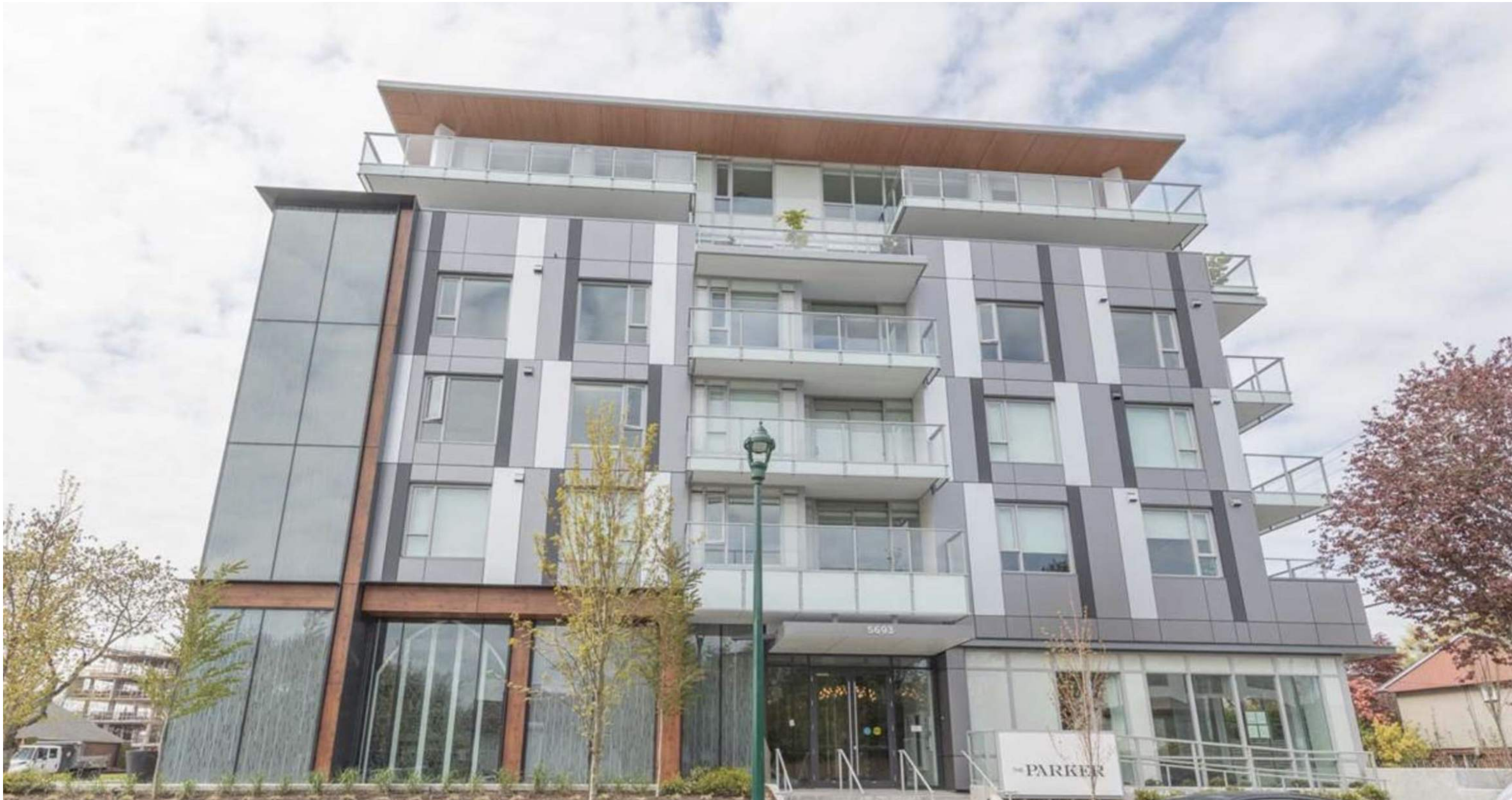
Aluminum and phenolic wood panels precedent
