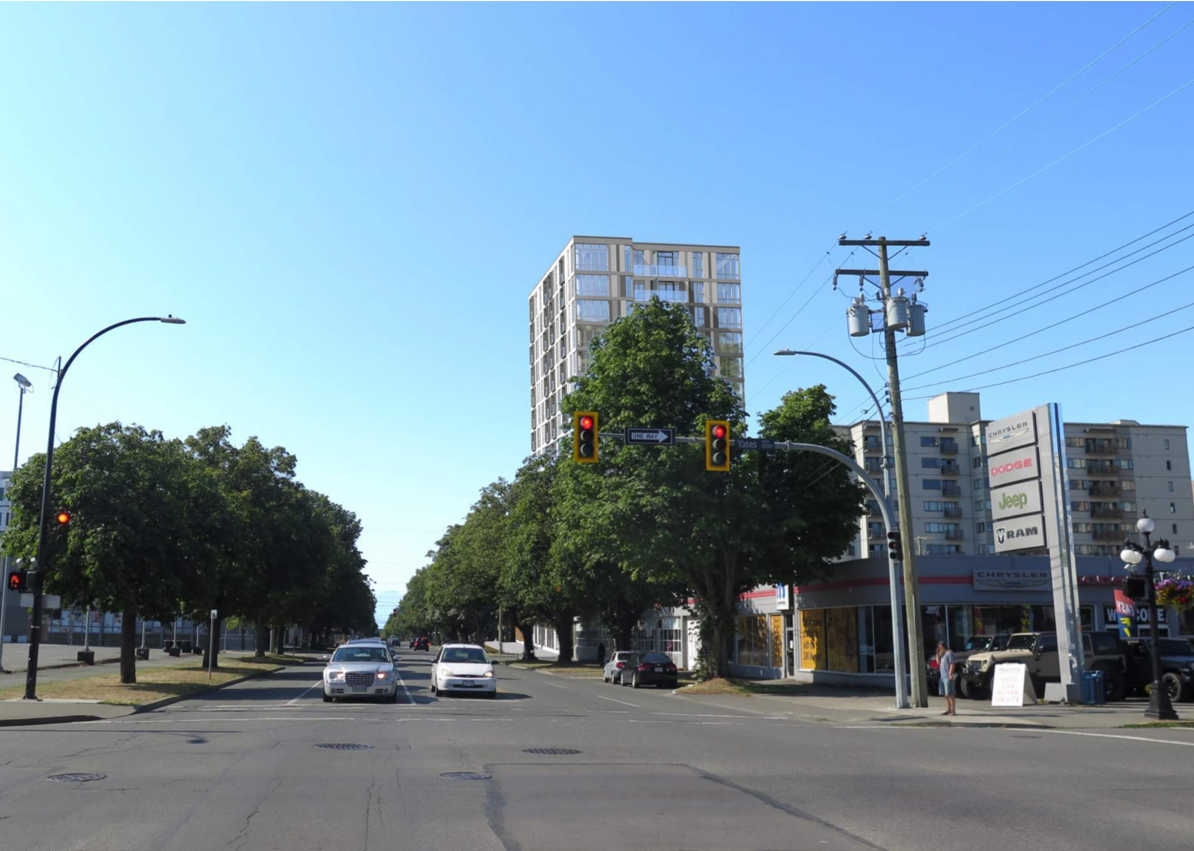
C Cook Street Looking South
