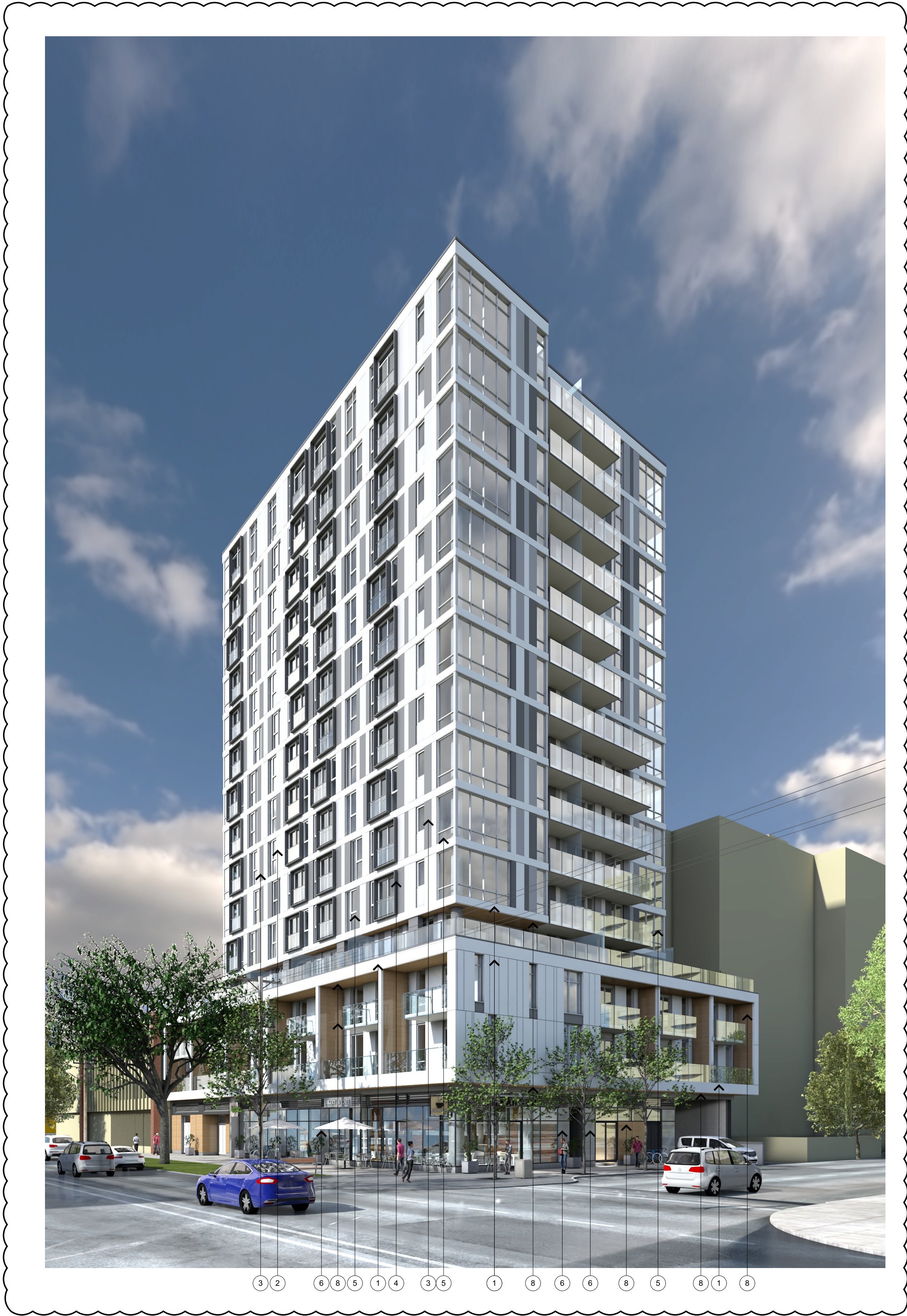
① Aluminum composite panel - Stac Bond Reference: STB-459 Color: Signal white - RAL 9003 Finish: Matte - Acabado
