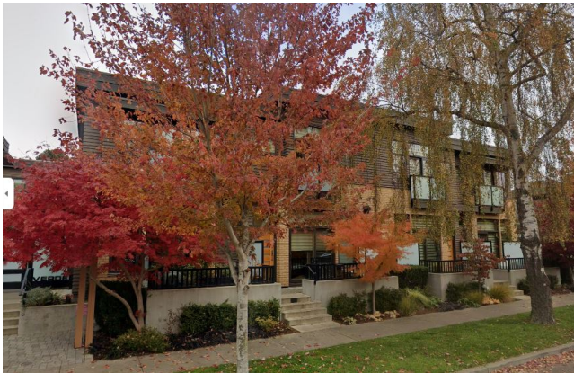
1020 Richardson Street (One lot over on same side of street)
