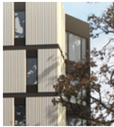
CONTEMPORARY & NEIGHBOURLY ARCHITECTURAL DESIGN
