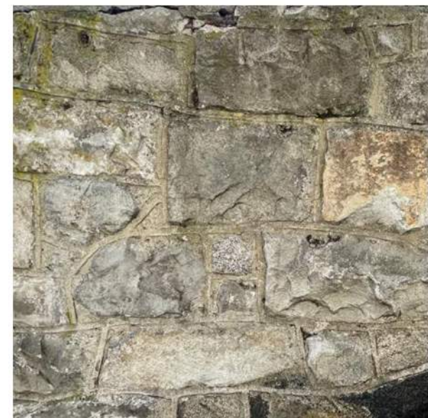
F2 EXISTING FENCING WALL
