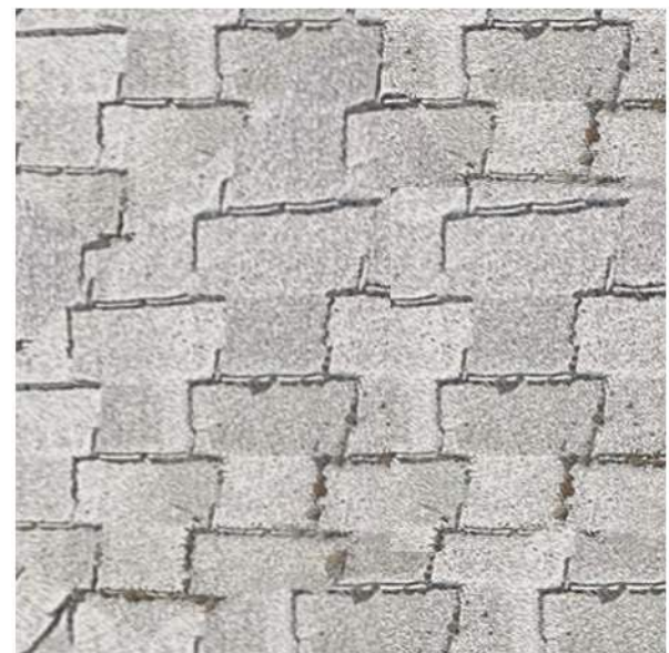
R1 EXISTING ROOF SHINGLES
