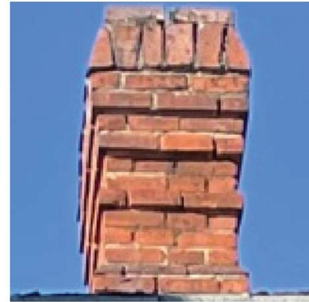
B1 EXISTING BRICK
