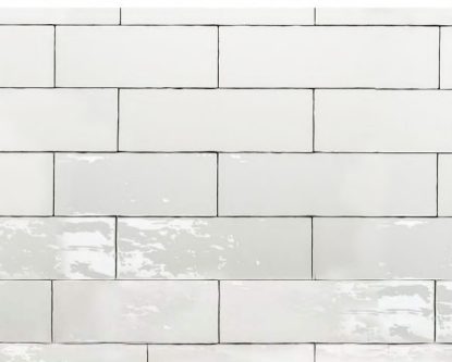
EXISTING WHITE GLAZED BRICK
