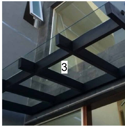
Glass/Metal Entrance Canopy
