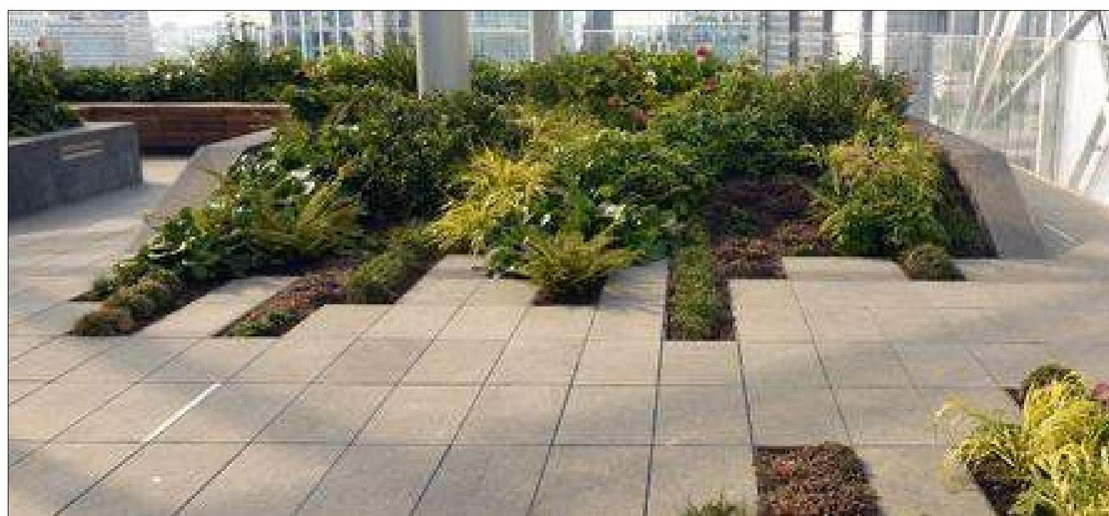
1) PRE-CAST CONCRETE PAVERS INTEGRATED WITH PLANTING
