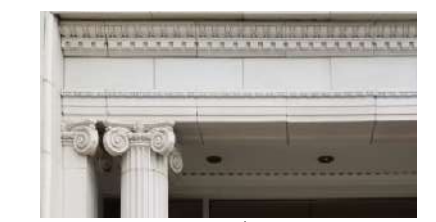
EXISTING STONE/PLASTER, ORNAMENTAL DETAILING.
