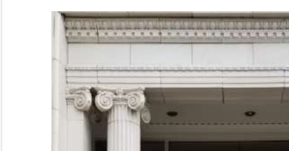
EXISTING STONE/PLASTER, ORNAMENTAL DETAILING.
