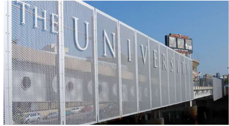
ROOF MECHANICAL SCREENING (PERFORATED METAL)
