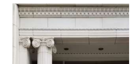
EXISTING STONE/PLASTER, ORNAMENTAL DETAILING.
