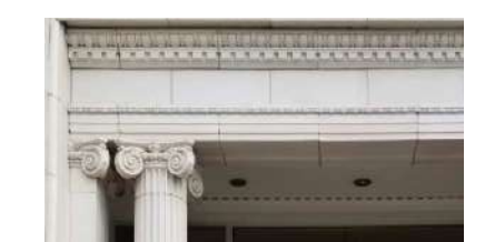
EXISTING STONE/PLASTER ORNAMENTAL DETAILING.
