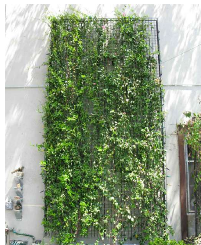
EAST SIDE, PARKADE WALL: WALLMOUNTED GREEN WALL PANELS GREENSCREEN 'ELEMENTS' MODULAR PANELS CUSTOM SIZE TO FIT, MOUNT PER MANUFACTURER SPECIFICATION
