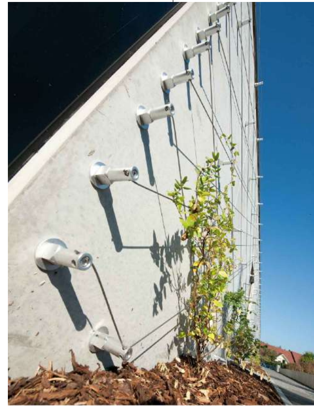
CABLE TRELLIS MOUNTED TO MASONRY WALL (SOUTH PL) CARL STAHL GREENCABLE SYSTEM OR SIMILAR W/ VINE PLANTED AT BASE
