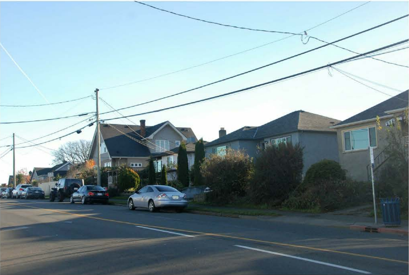
03. Burnside Rd E- looking south
