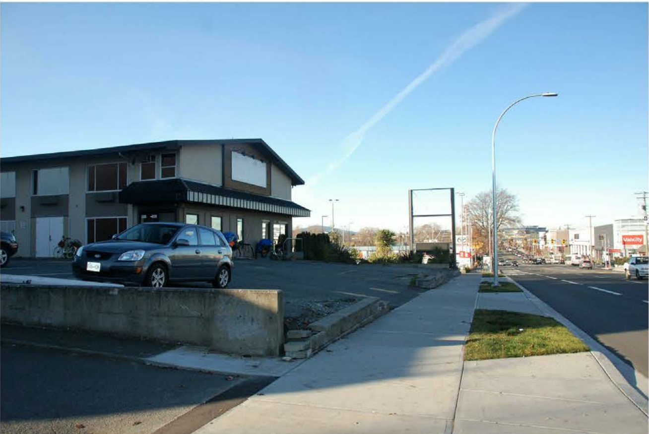
07. Site from Douglas St- looking north
