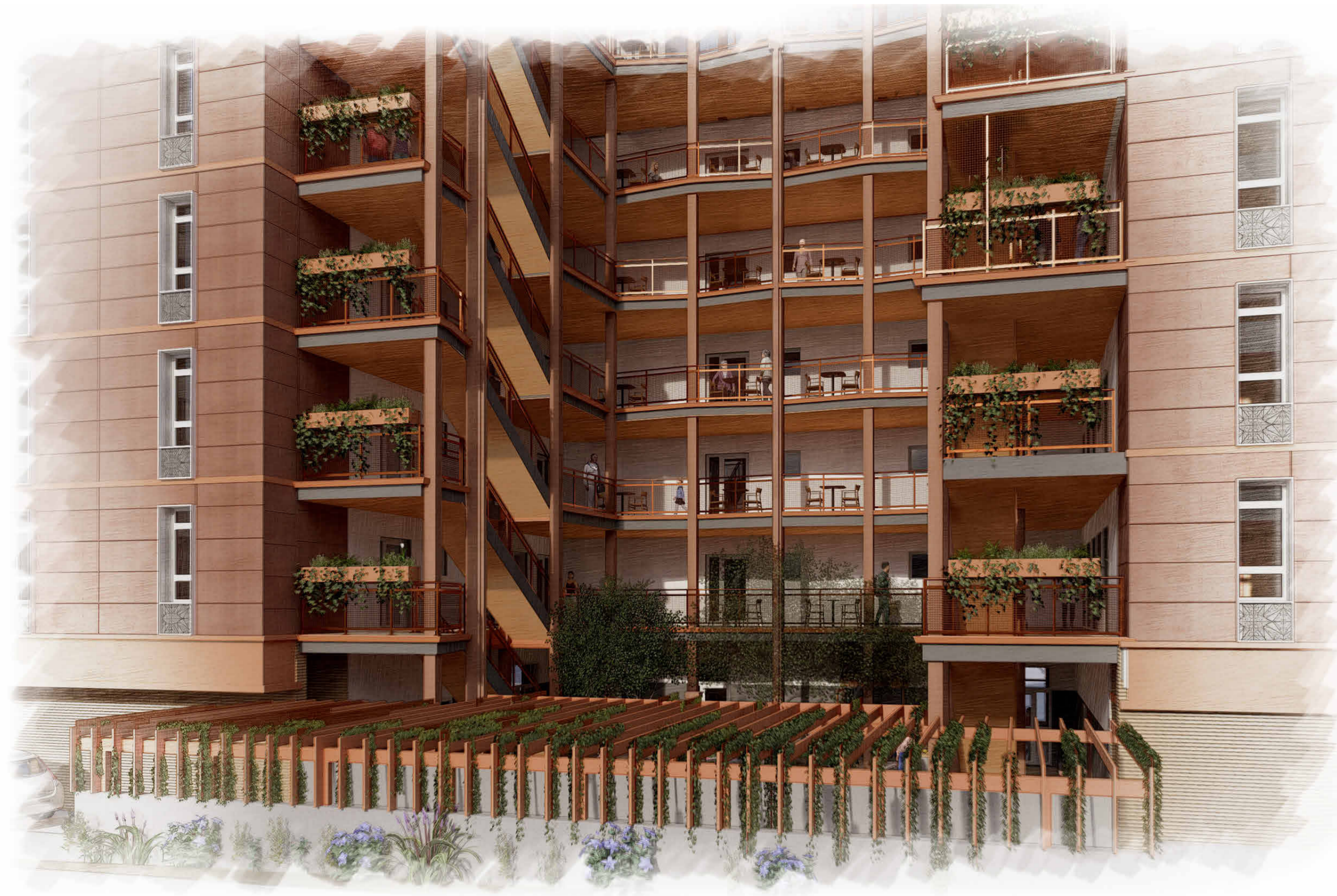
COURTYARD LOOKING NORTH
