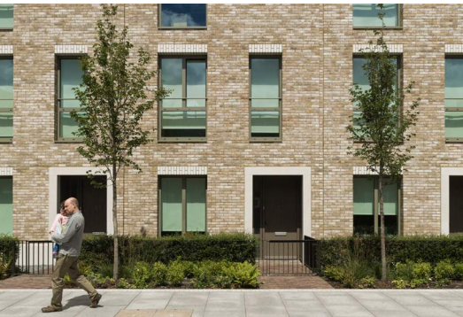
Active Residential - front doors
