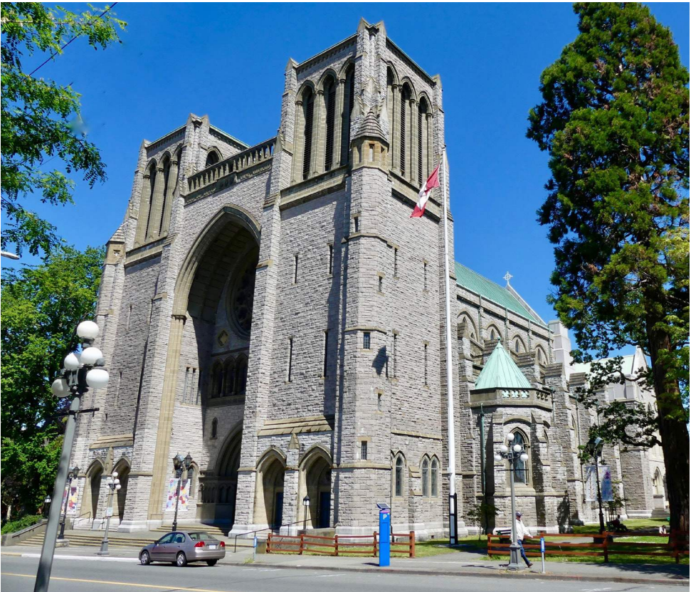
Current South-East view
