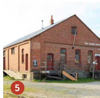
Stores building, view from east
