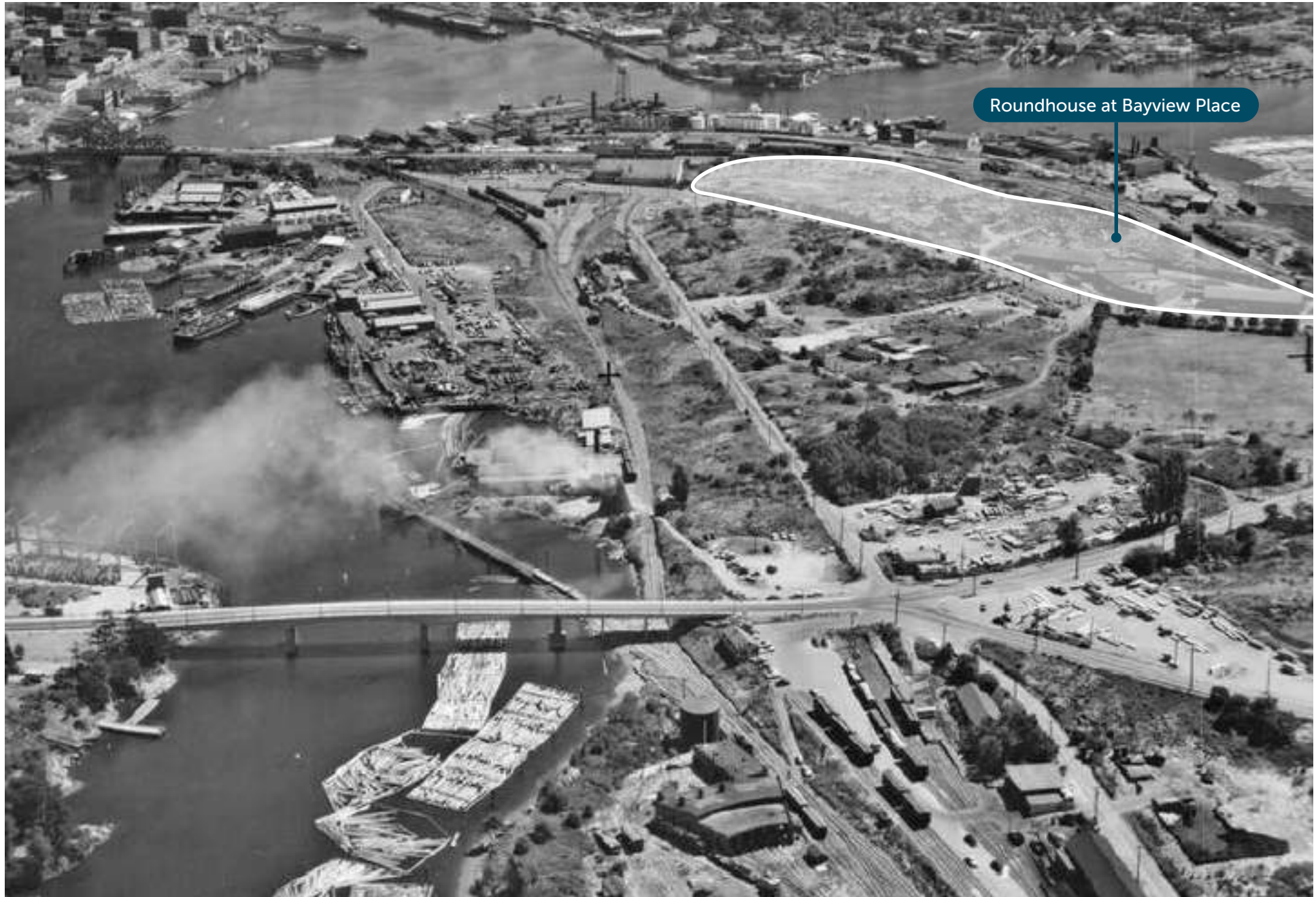
Aerial Photo of Roundhouse at Bayview Place Site
