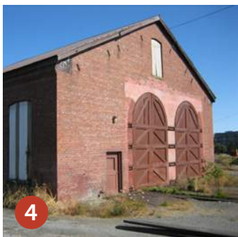
Car shop, view from west
