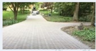
**Benefits:** Reduce runoff volume and improve water quality by infiltrating and treating stormwater while still providing a hard, drivable surface.
