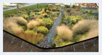
**Benefits:** Reduce runoff volume and increase water quality by capturing, detaining, treating, and conveying stormwater.
