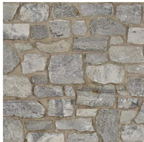
ST COURSED STONE RECLAIMED MATCH EXISTING PATTERN
