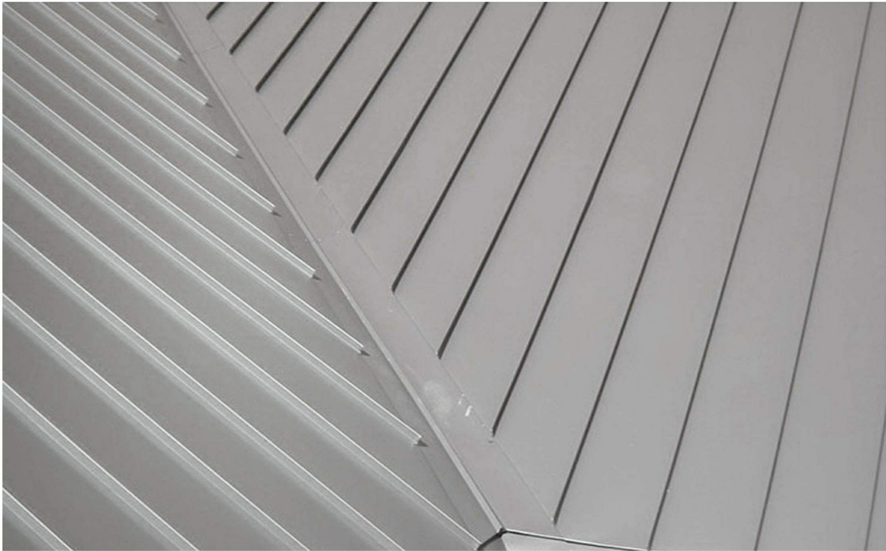
ROOFING: STANDING SEAM METAL ROOF - ZINC COLOUR
