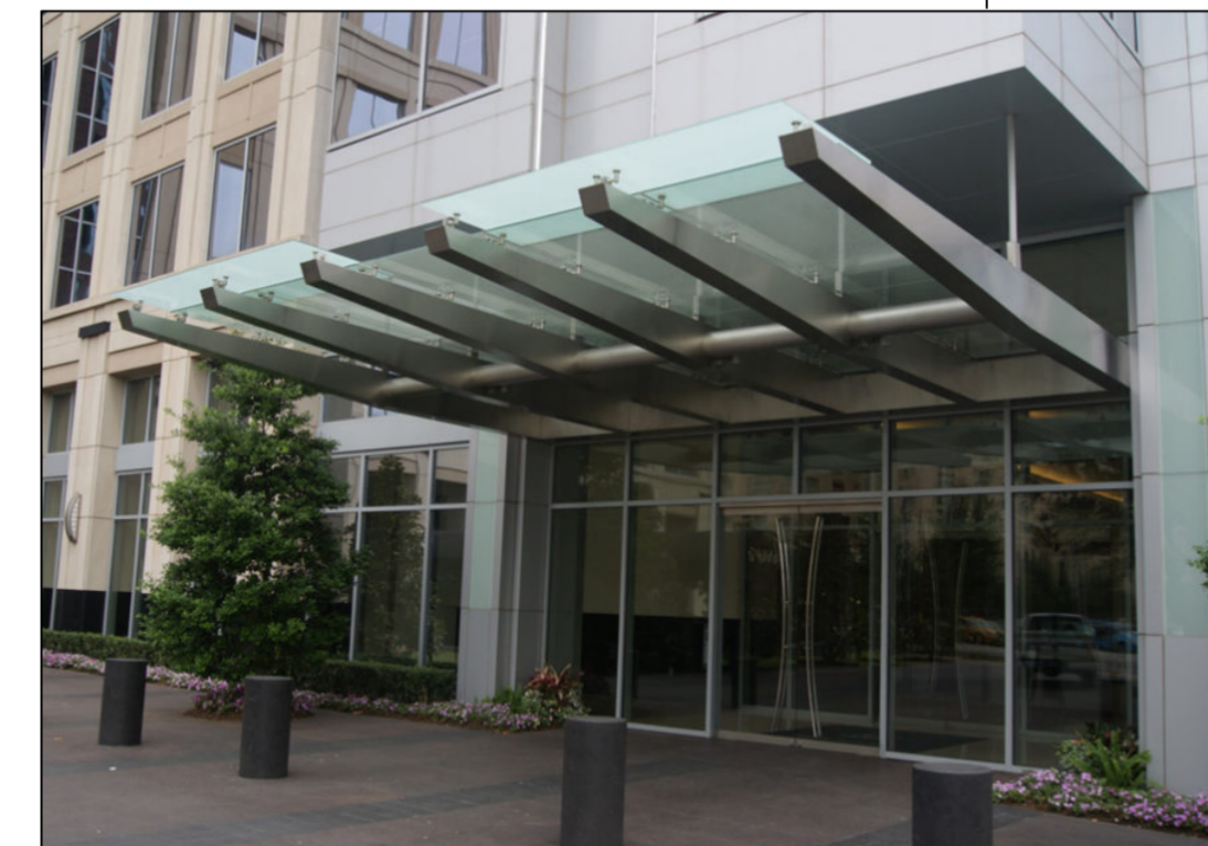
Steel and glass canopy
