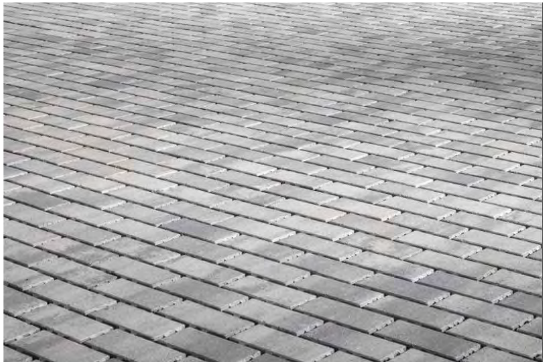
2 BELGARD AQUALINE PERMEABLE PAVER L3 NTS
