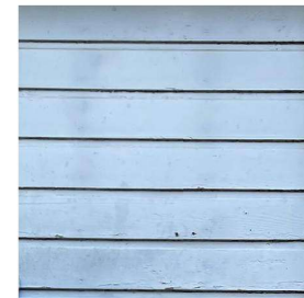
S1 EXISTING CHANNEL RUSTIC SIDING
