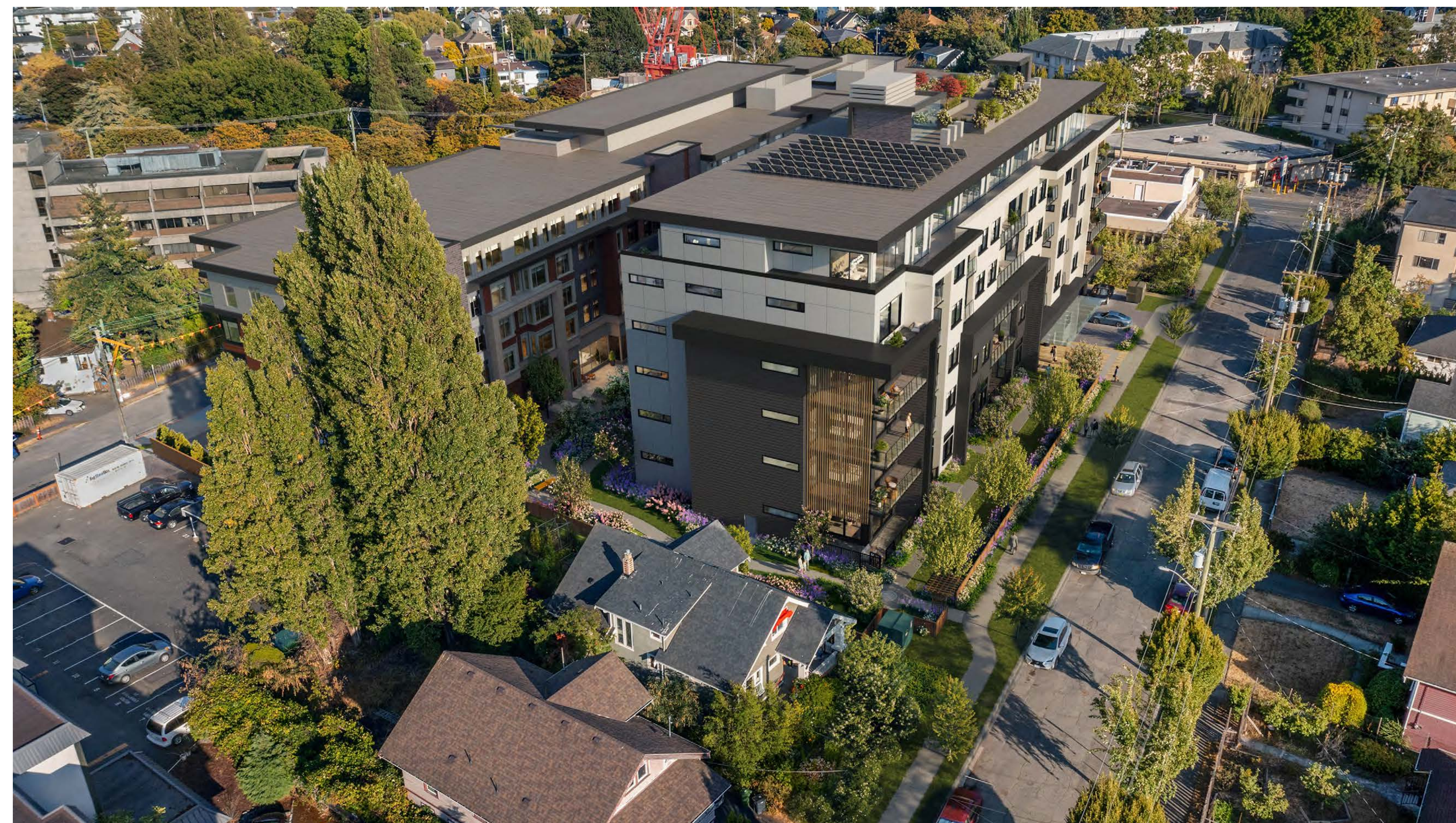
Aerial View - Looking South East from Ashgrove Street Phase 1 in Background
