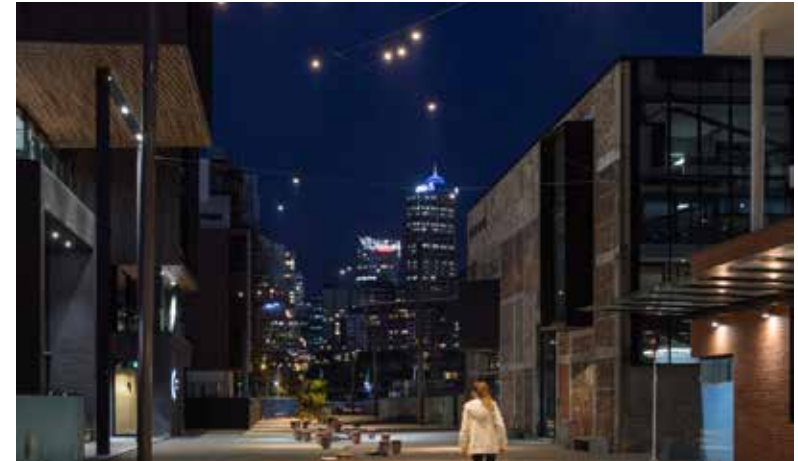
Combination of catenary, pedestrian scale, soffit and plaza lighting
