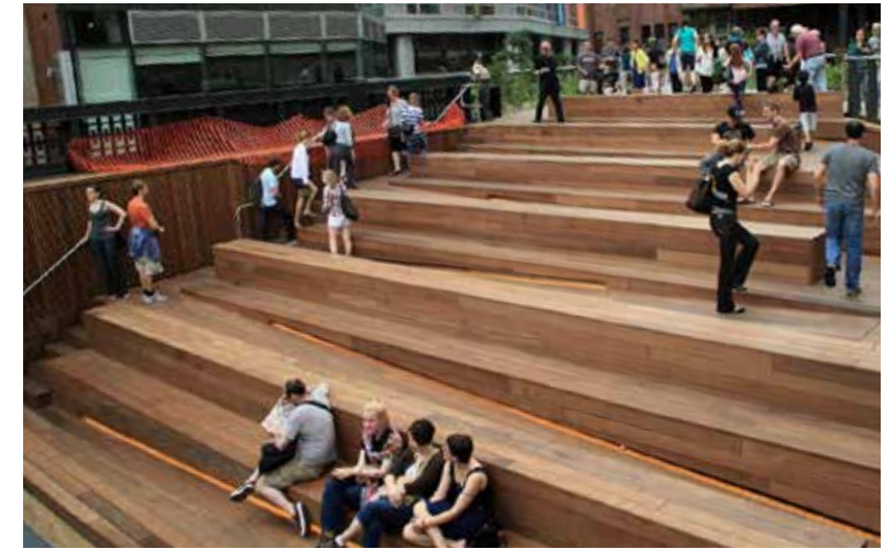
Terraced seat steps with accessibility ramp incorporated
