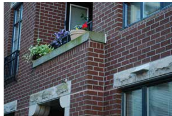
Change in material pattern to emphasize building elements, in this case windows and entrances.
