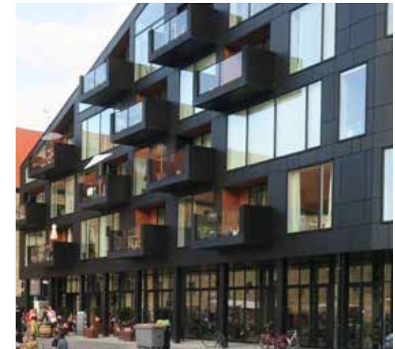
Projecting balconies provide interest above the street level
