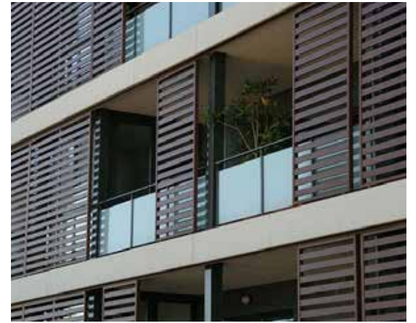
Sun shading screens integrated into façade
