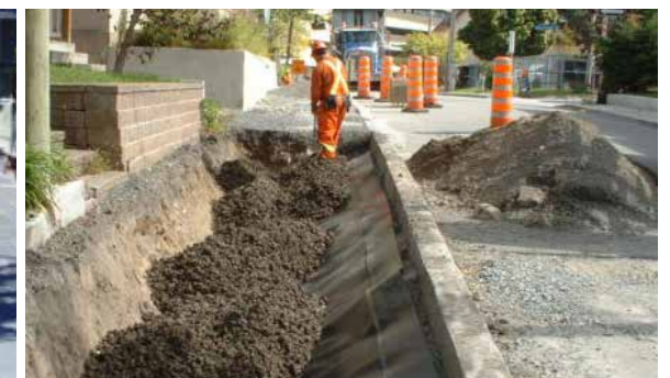
Structural soil installation
