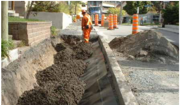
Structural soil installation
