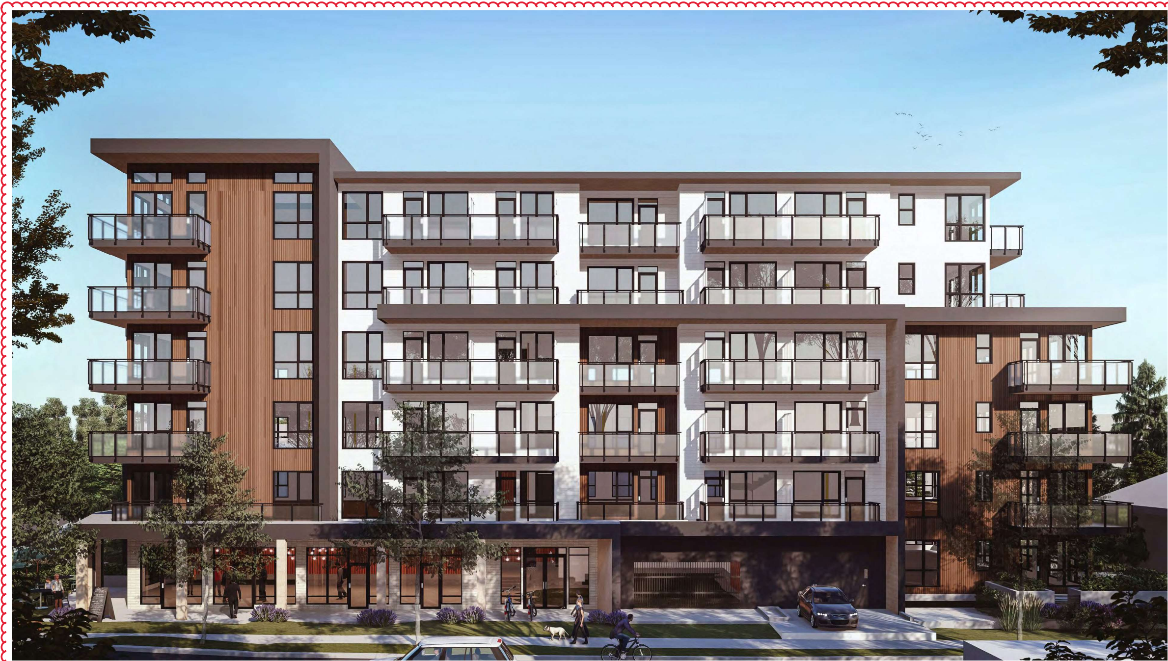
West Elevation - Davie St
