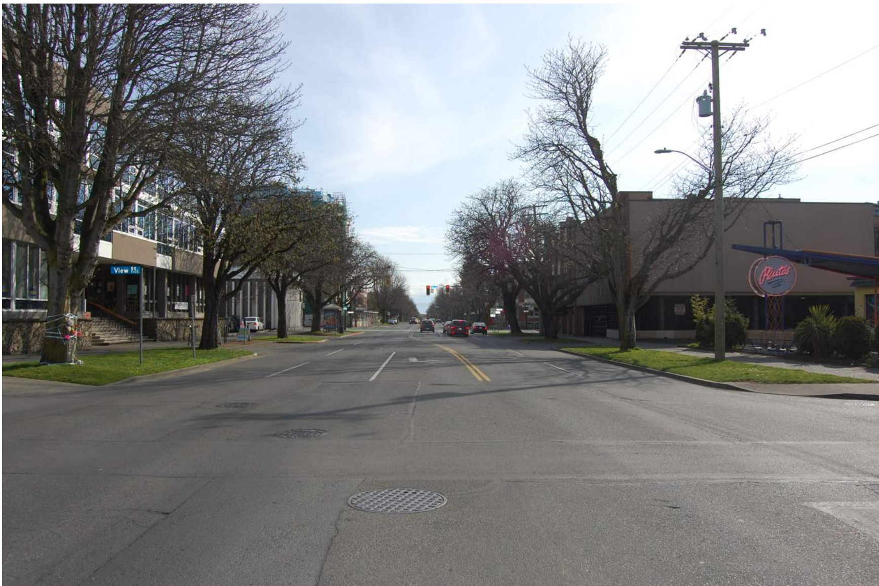
2. Cook Street Looking North
