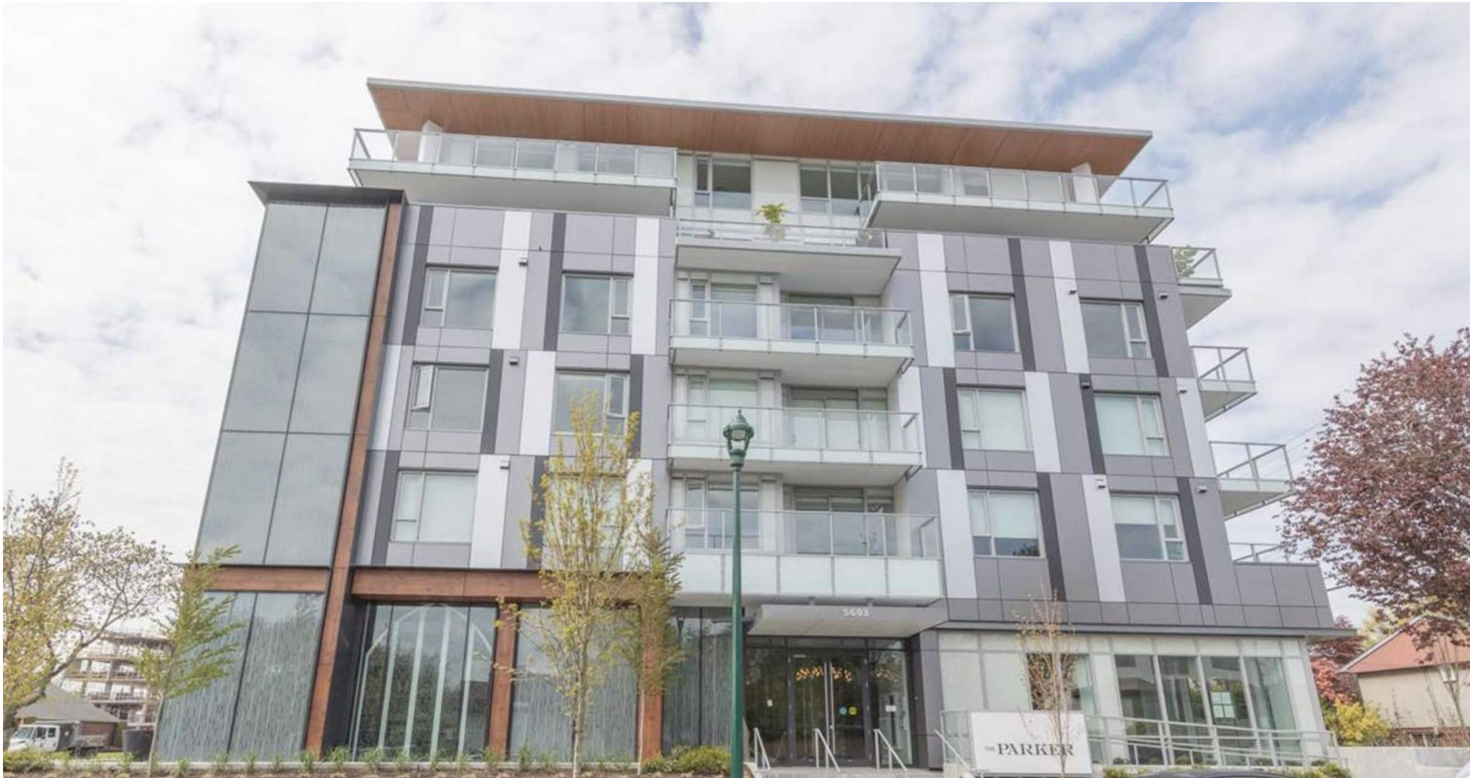
Aluminum and phenolic wood panels precedent
