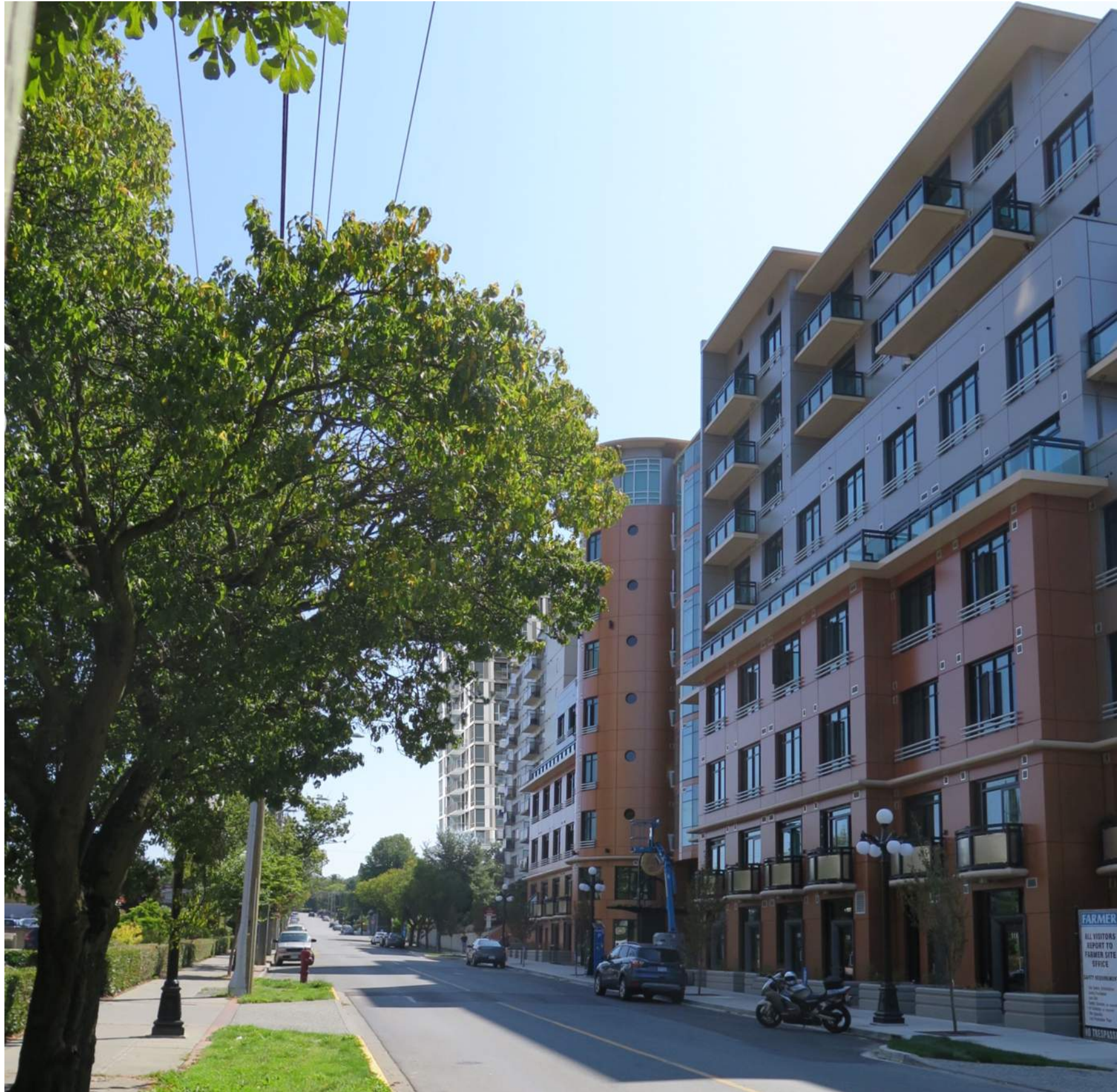
B View Street Looking East
