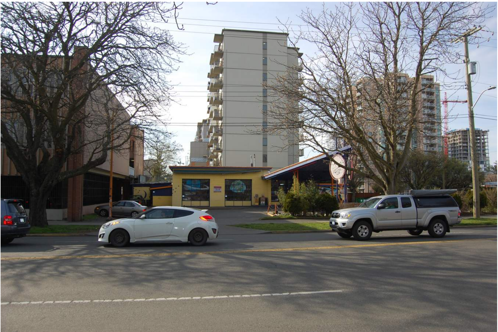
3. Site along Cook Street
