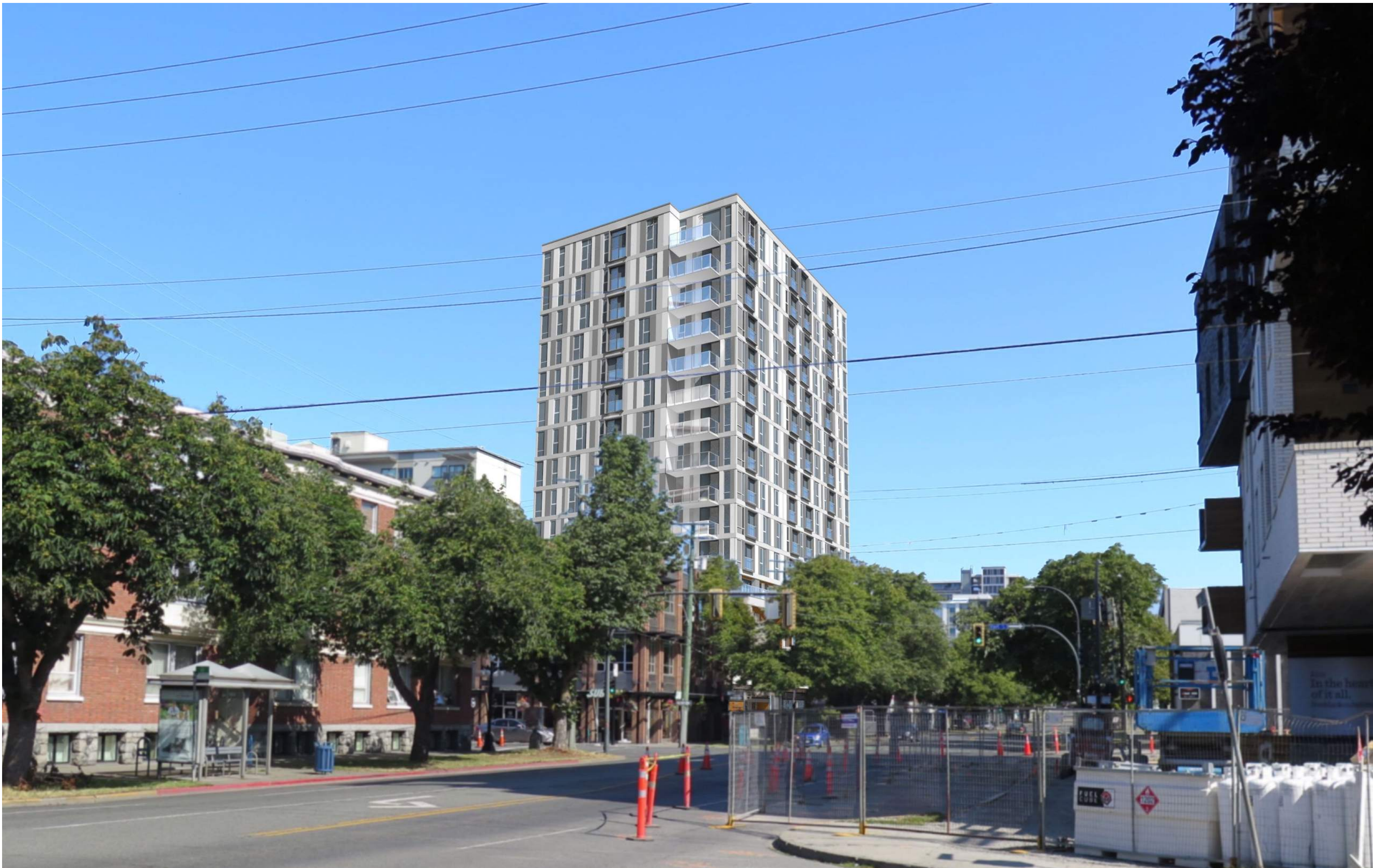
A Cook Street Looking North
