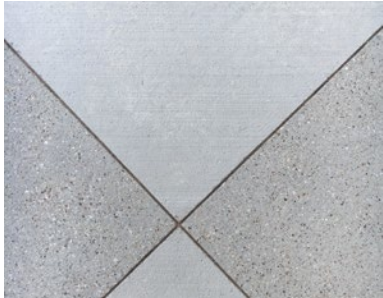
Cast-in-place Concrete (sawcut, non-slip)
