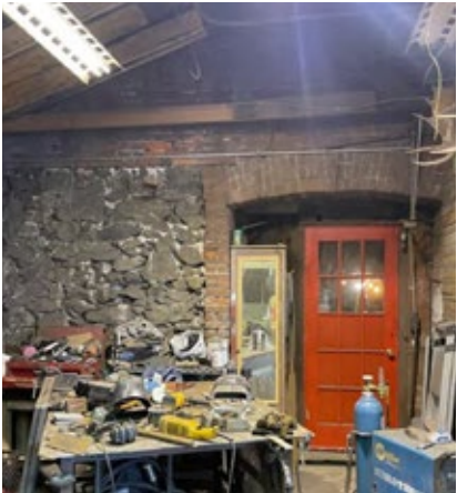
2021, Lower Level West Elevation
