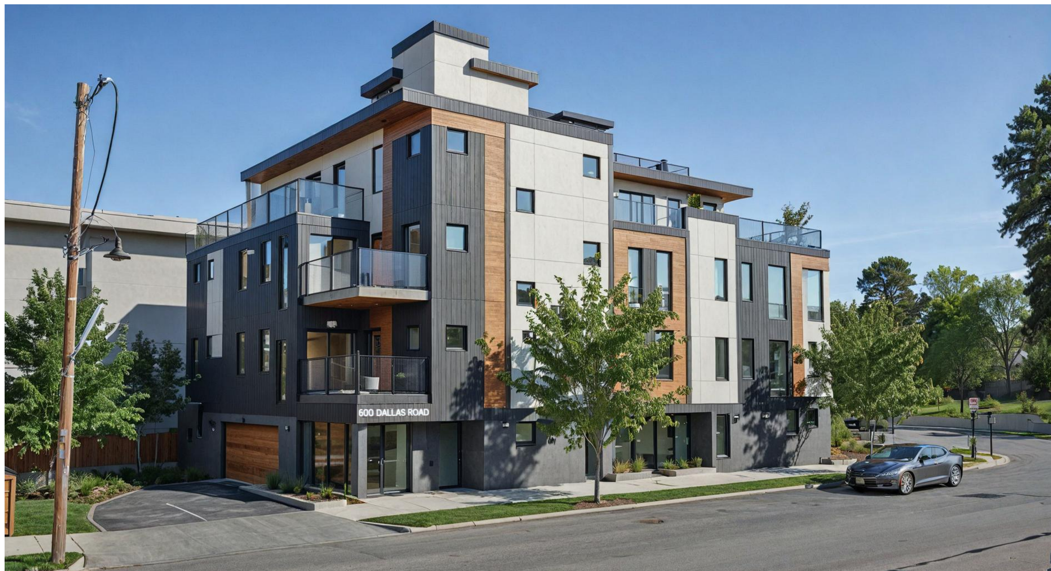
VIEW OF PROJECT FROM GOVERNMENT STREET
