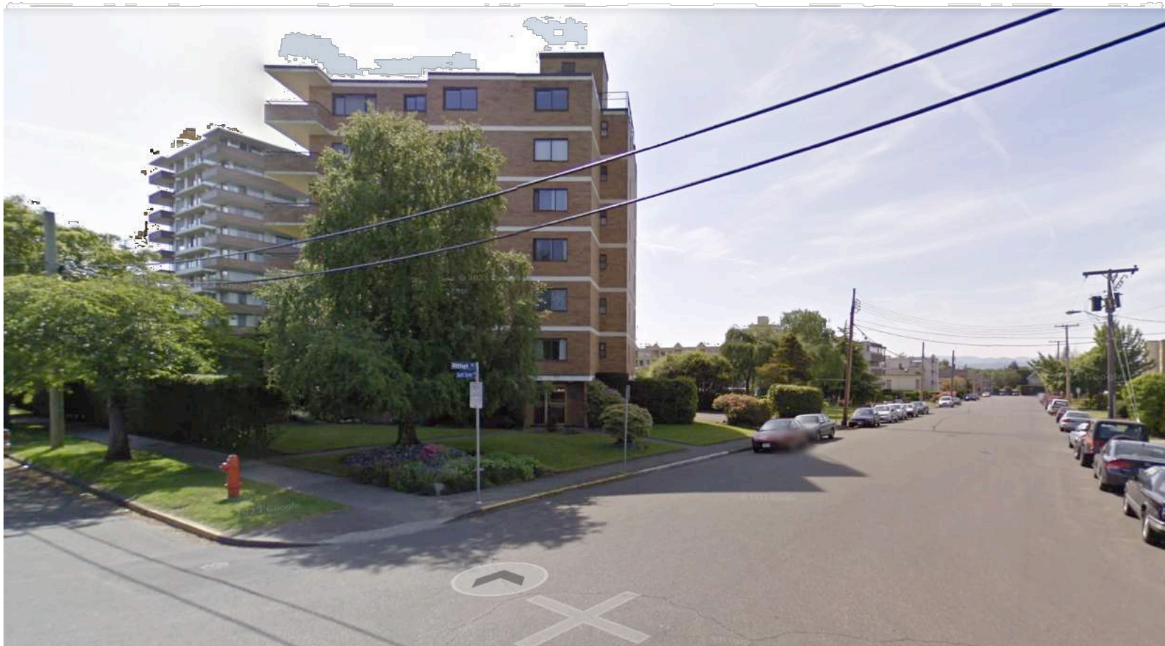
4 RITHET ST - EXISTING BUILDINGS - WESTWARD VIEW
