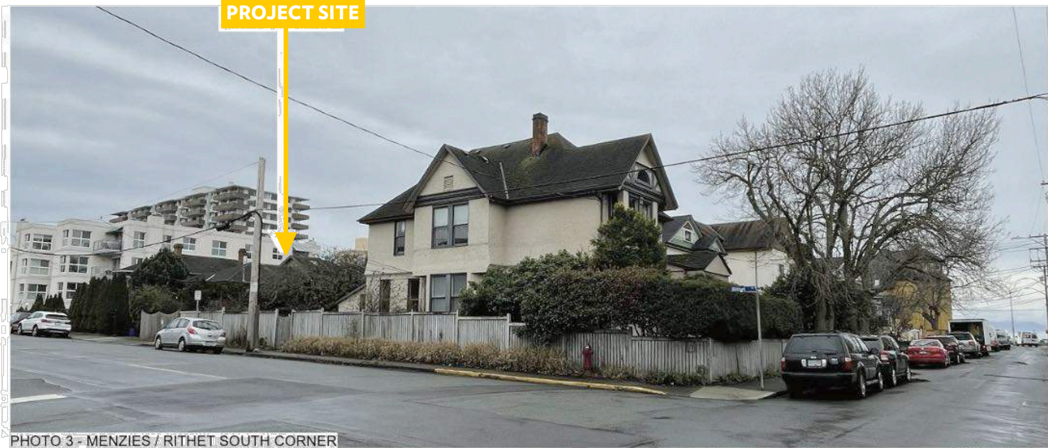
PHOTO 3 - MENZIES / RITHET SOUTH CORNER
