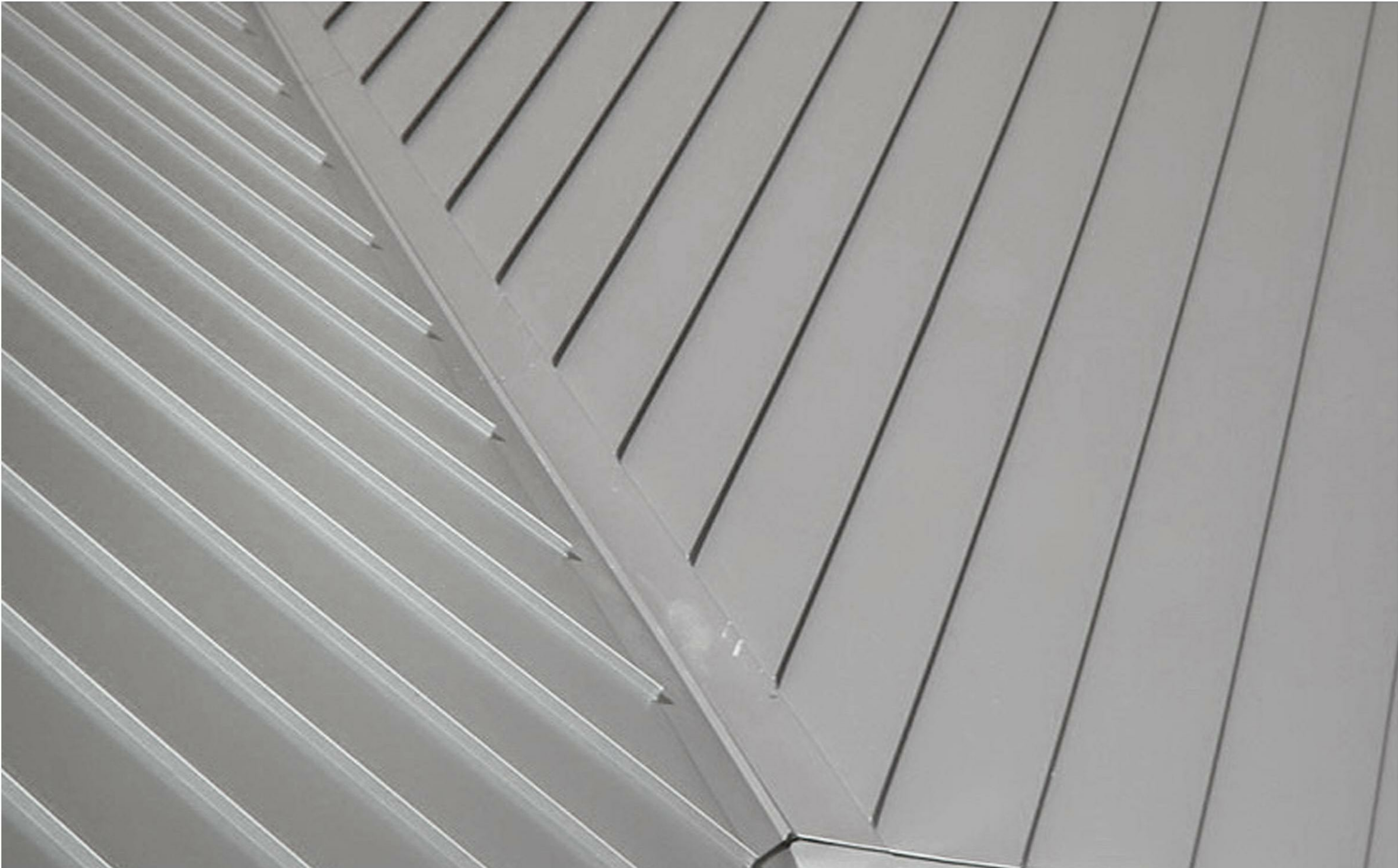
ROOFING: STANDING SEAM METAL ROOF - ZINC COLOUR
