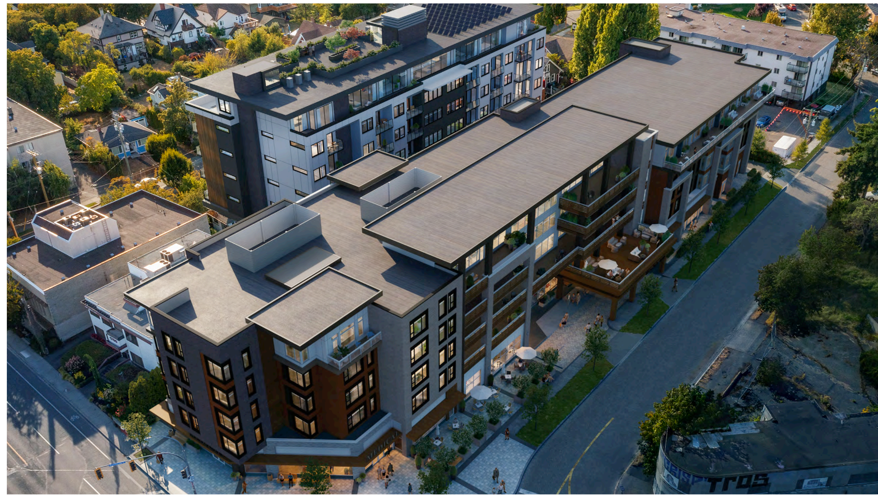
Aerial View - Looking West from Richmond Road Phase 1 in Foreground
