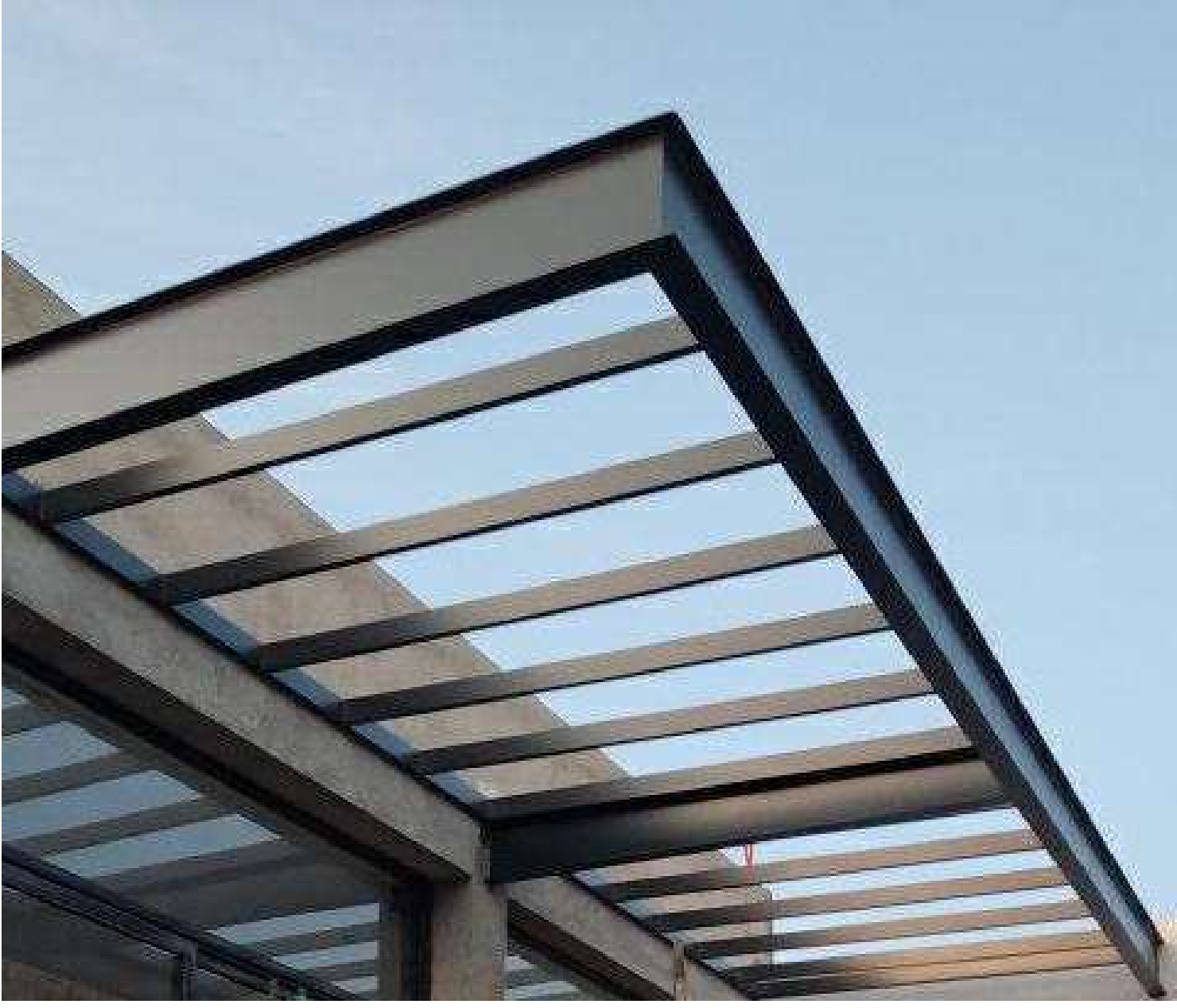
BLACK PAINTED STEEL CANOPY W/ LAMINATED GLAZING
