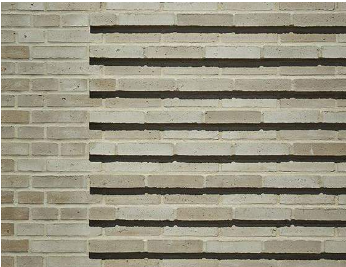
HORIZONTAL BRICK REVEAL DETAILING
