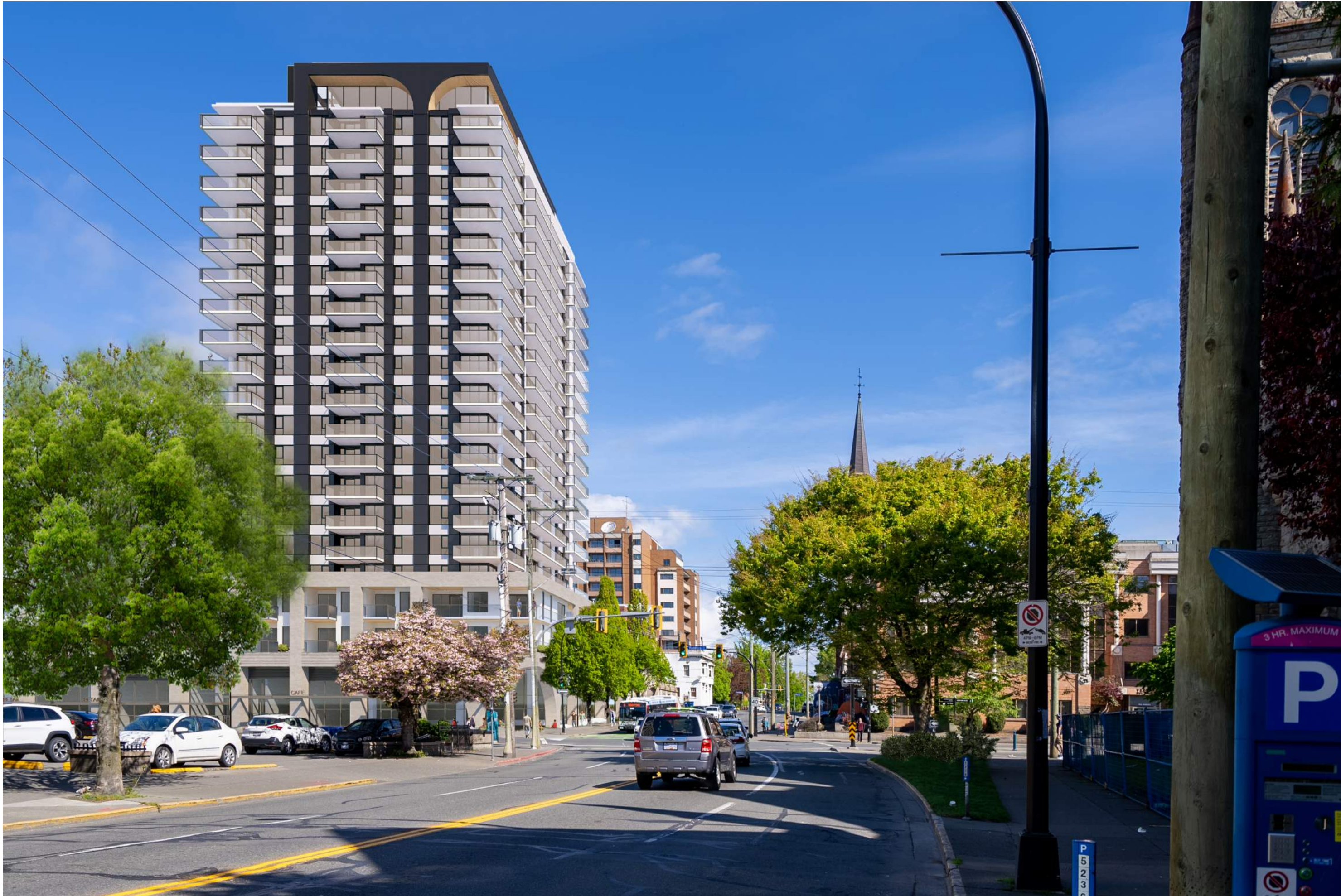
LOOKING NORTH ON QUADRA ST.
