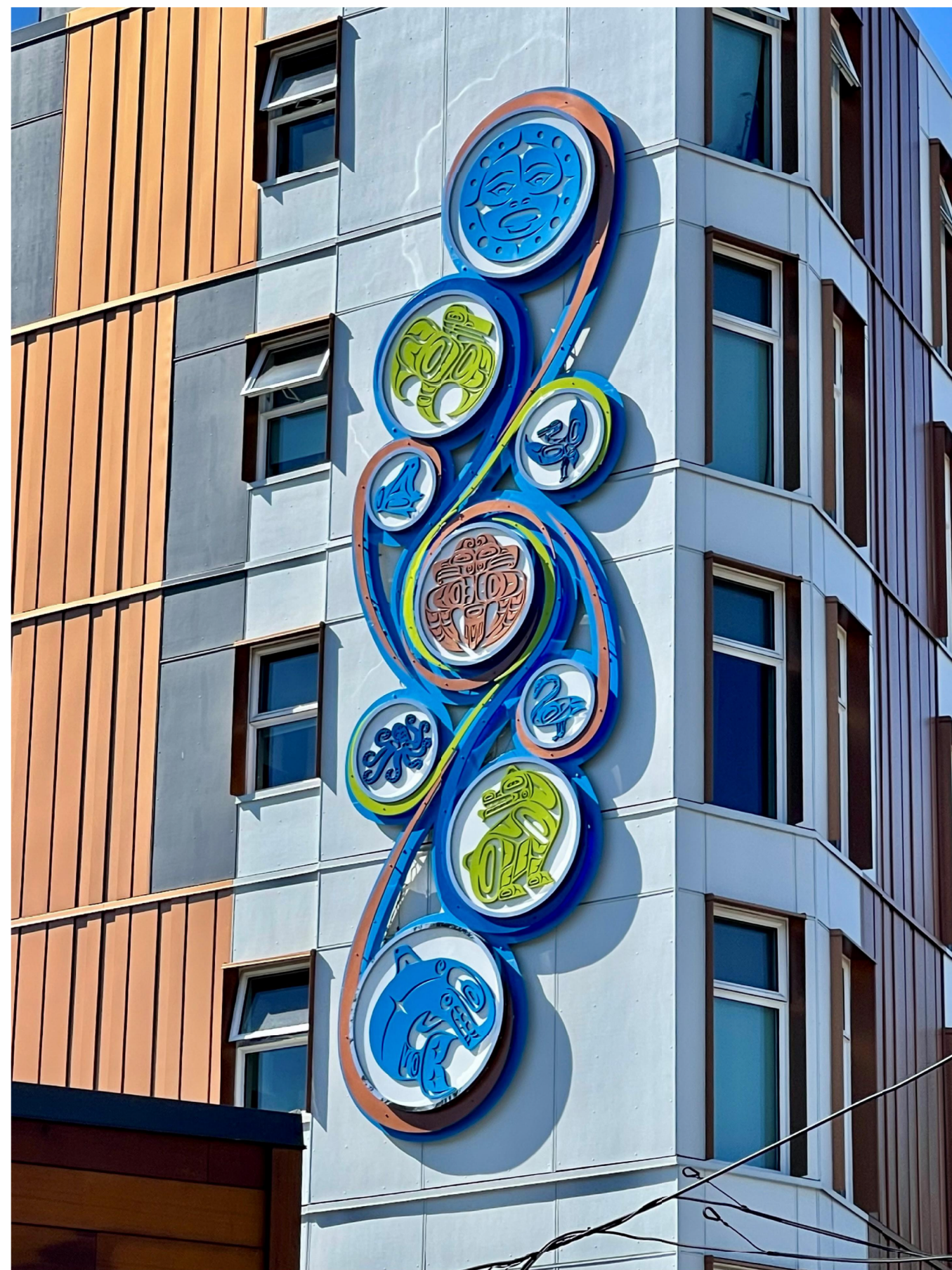
LIFE ENERGY - 2020 (M'AKOLA HOUSING SOCIETY MAIN OFFICE)
