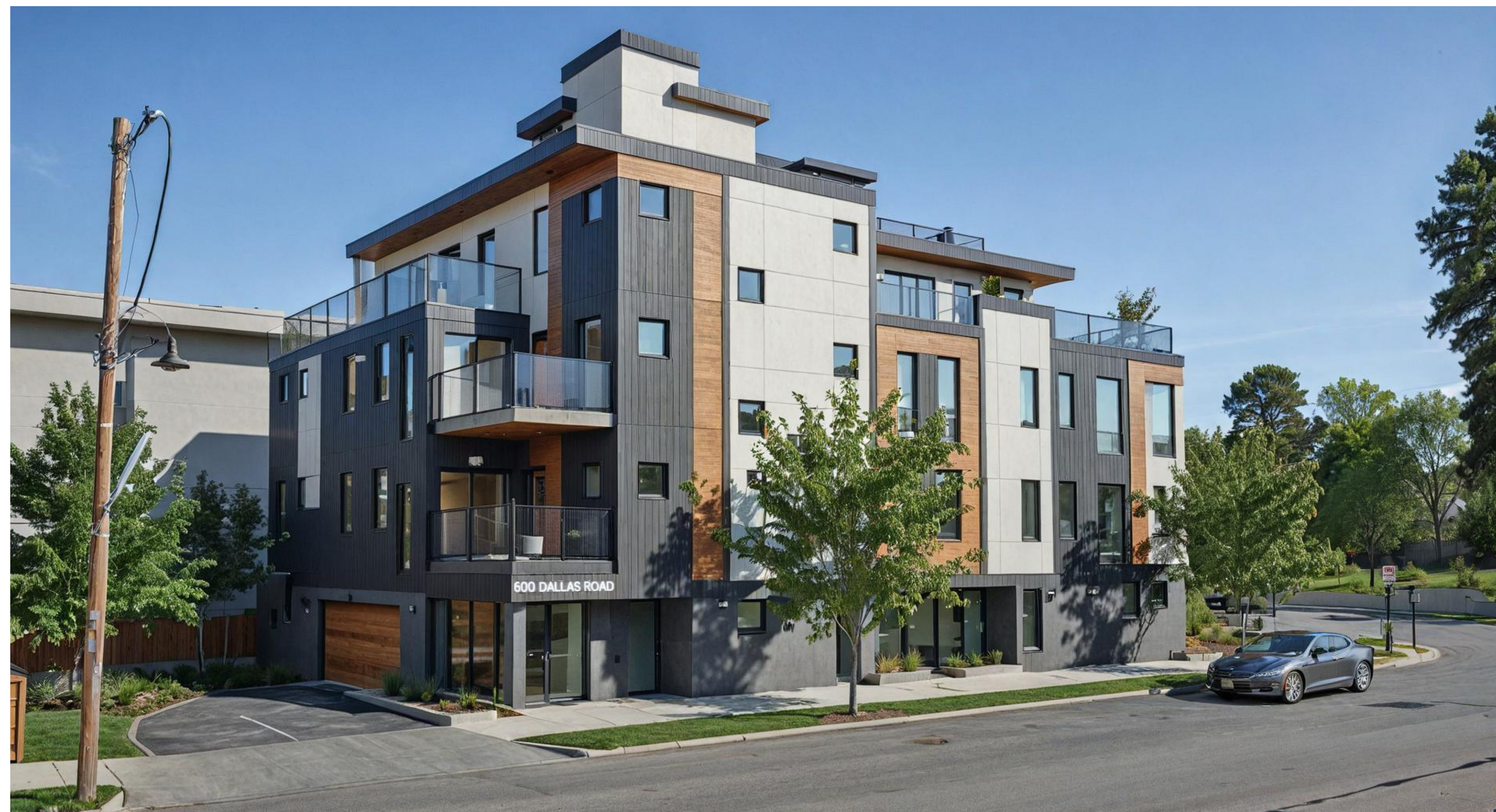
VIEW OF PROJECT FROM GOVERNMENT STREET
