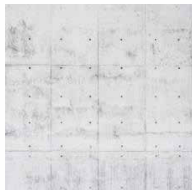
(4) ARCHITECTURAL CONCRETE COLOUR: WHITE
