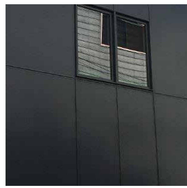
(3) ALUMINUM SANDWICH PANELS COLOUR: CHARCOAL
