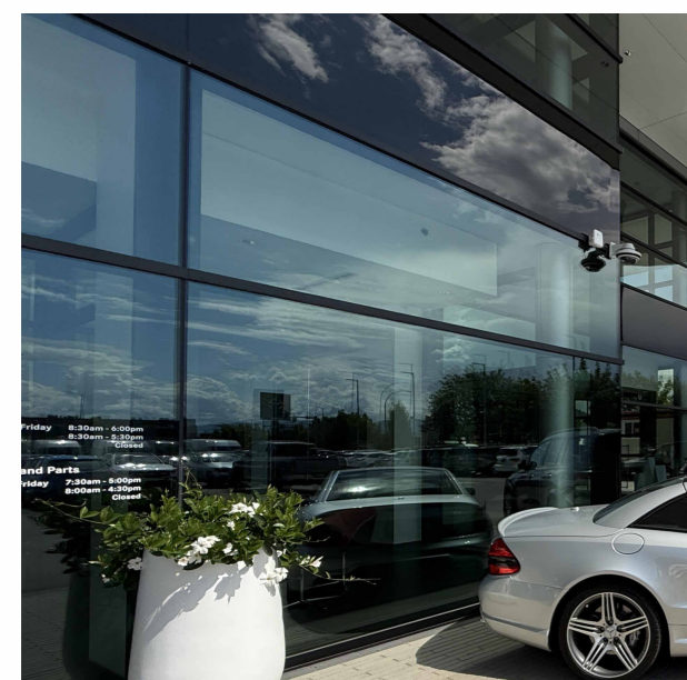
(1) ALUMINUM STOREFRONT WINDOW/DOOR COLOUR: CHARCOAL
