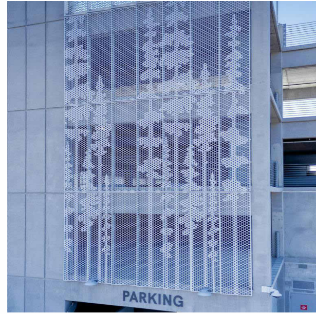
(5) PERFORATED GRAPHIC PANEL COLOUR: WHITE
