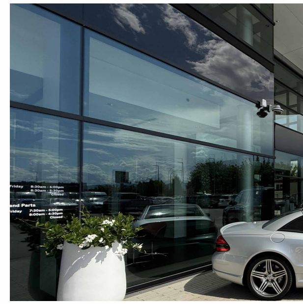
(1) ALUMINUM STOREFRONT WINDOW/DOOR COLOUR: CHARCOAL
