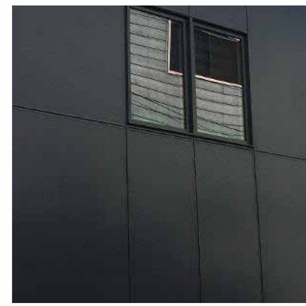
(3) ALUMINUM SANDWICH PANELS COLOUR: CHARCOAL
