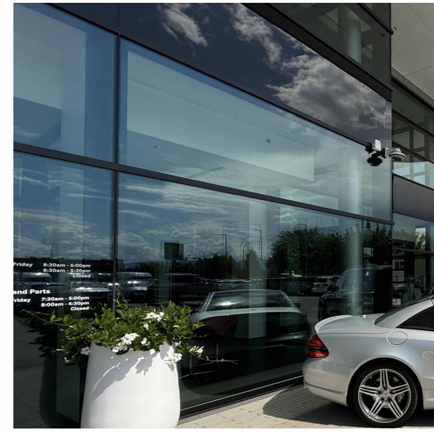
(1) ALUMINUM STOREFRONT WINDOW/DOOR COLOUR: CHARCOAL
