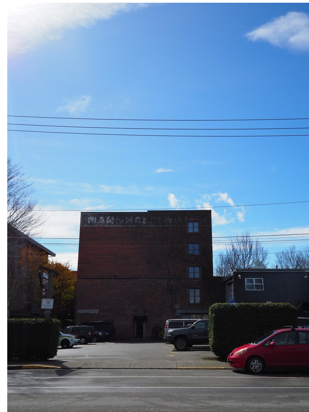
Image Reference # C5 Description: North Facade of Biggerstaff Building
