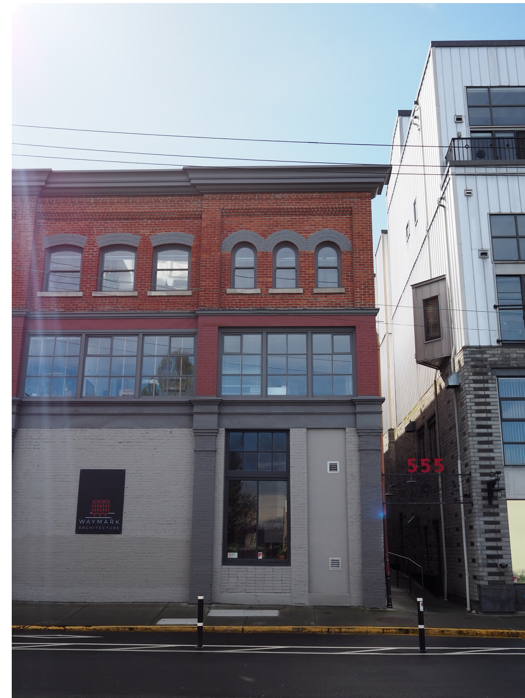
Image Reference # C2 Description: Commercial Building, Two Storey Residential
