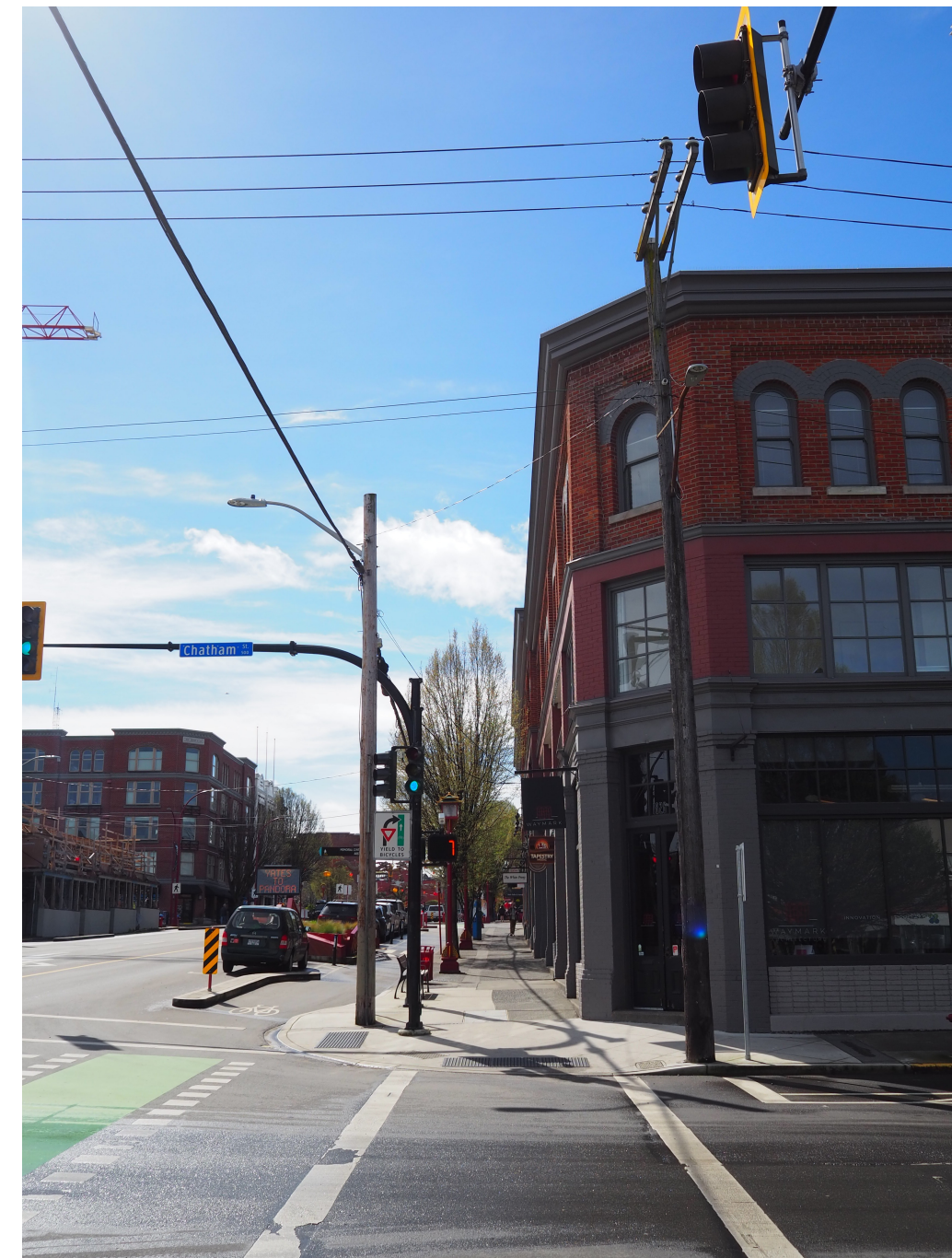
Image Reference # C1 Description: Commercial Building, Two Storey Residential
