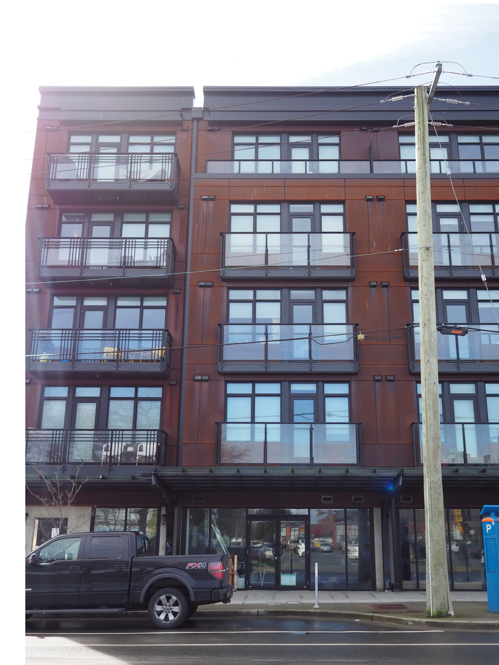
Image Reference # C6 Description: Adjacent Residential Building, Ironworks
