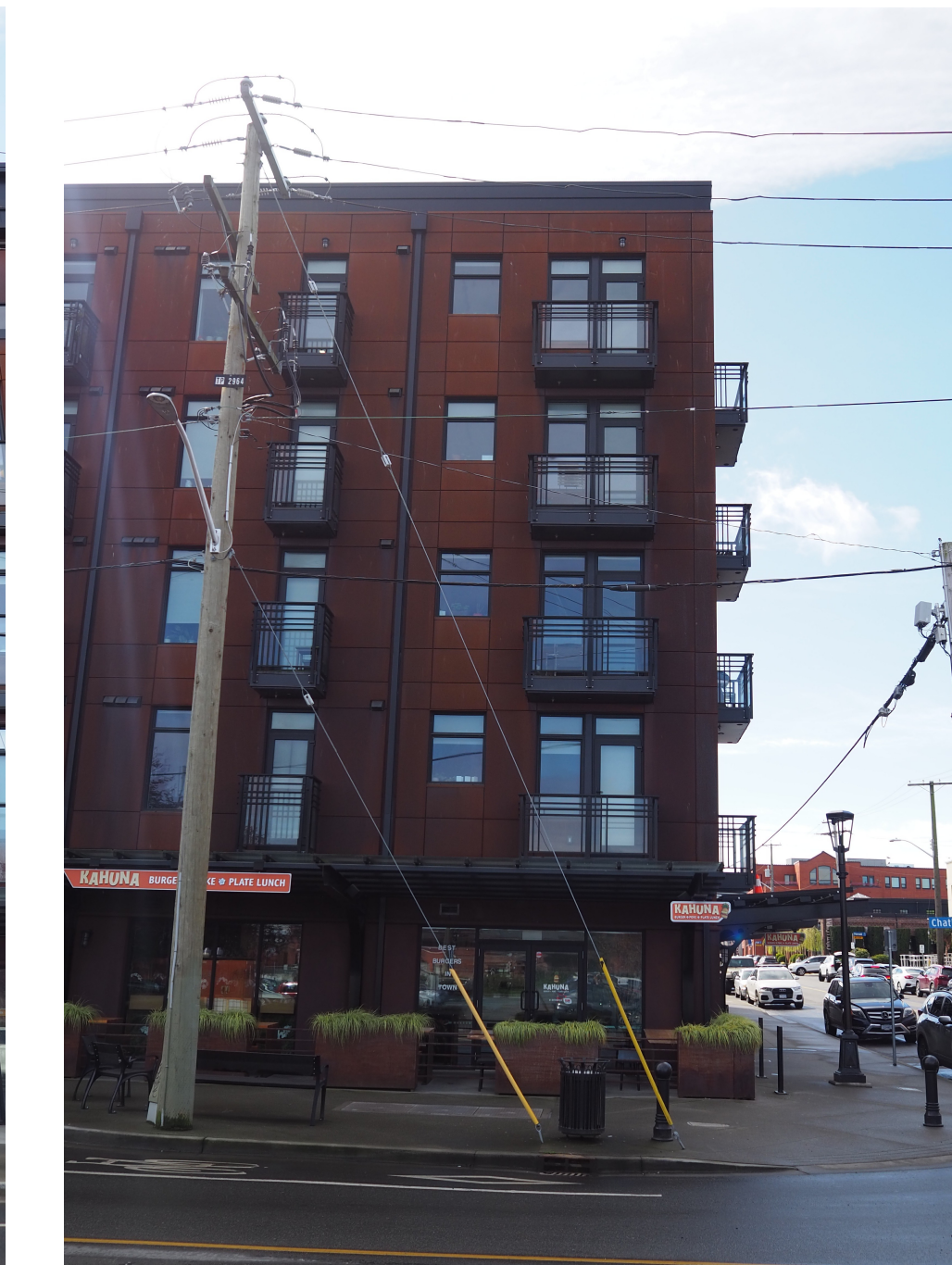
Image Reference # C7 Description: Adjacent Residential Building, Ironworks
