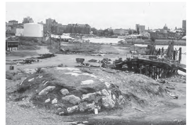
Site looking east, 1983
