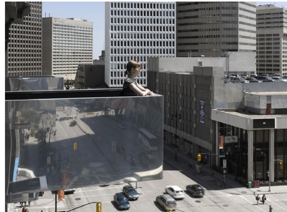
The Avenue on Portage 5468796 Architecture Winnipeg
