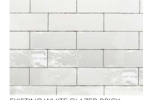
EXISTING WHITE GLAZED BRICK
