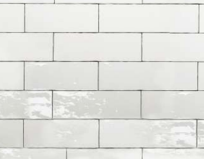
EXISTING WHITE GLAZED BRICK
