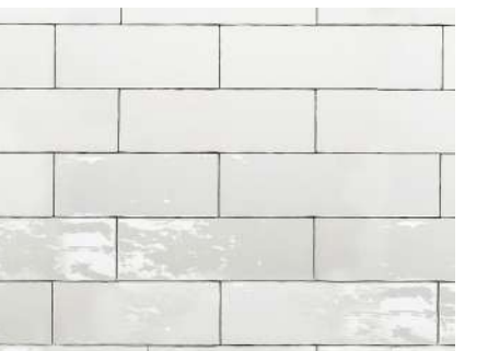
EXISTING WHITE GLAZED BRICK
