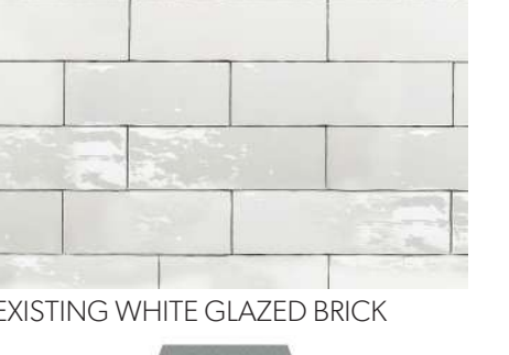
EXISTING WHITE GLAZED BRICK
