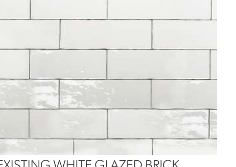
EXISTING WHITE GLAZED BRICK
