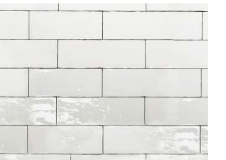
EXISTING WHITE GLAZED BRICK
