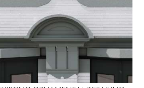
EXISTING ORNAMENTAL DETAILING RESTORED TO HERITAGE COLOUR PALETTE
