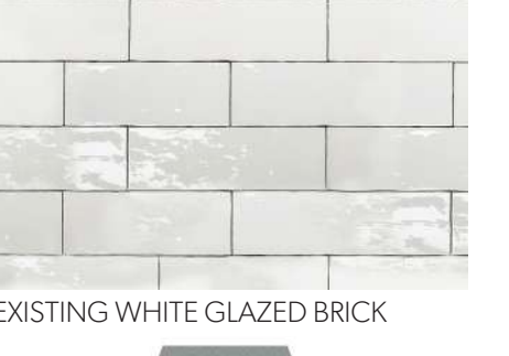
EXISTING WHITE GLAZED BRICK
