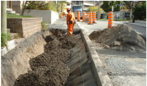
Structural soil installation
