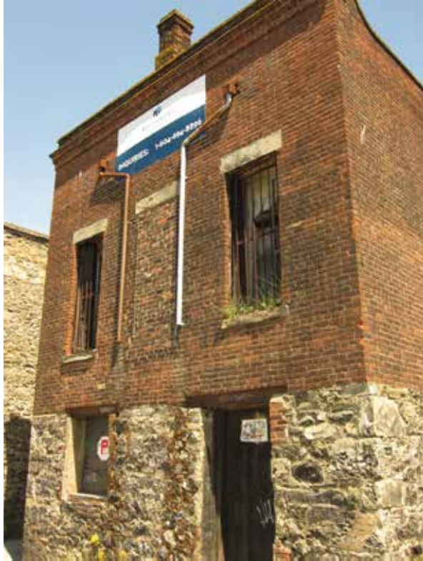
Current rear elevation of the Caire & Grancini Warehouse.
