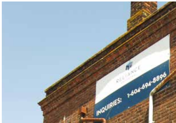
Above: Corbelled brick cornice on rear façade.
