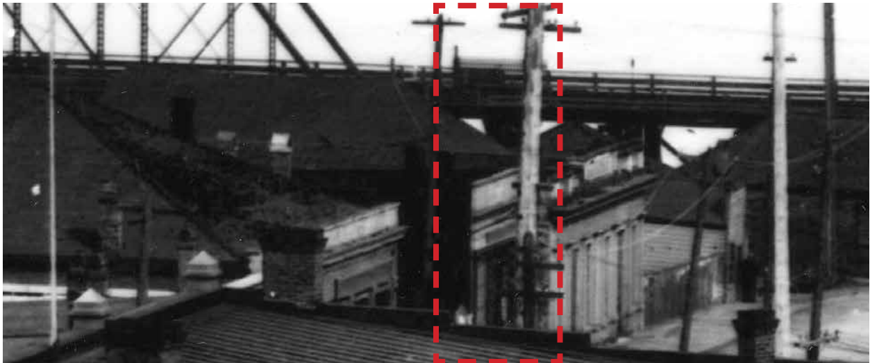
Oblique view of the front façade - Caire & Grancini Warehouse, one part of the Northern Junk Buildings - 1890s [BCA F-09561]
