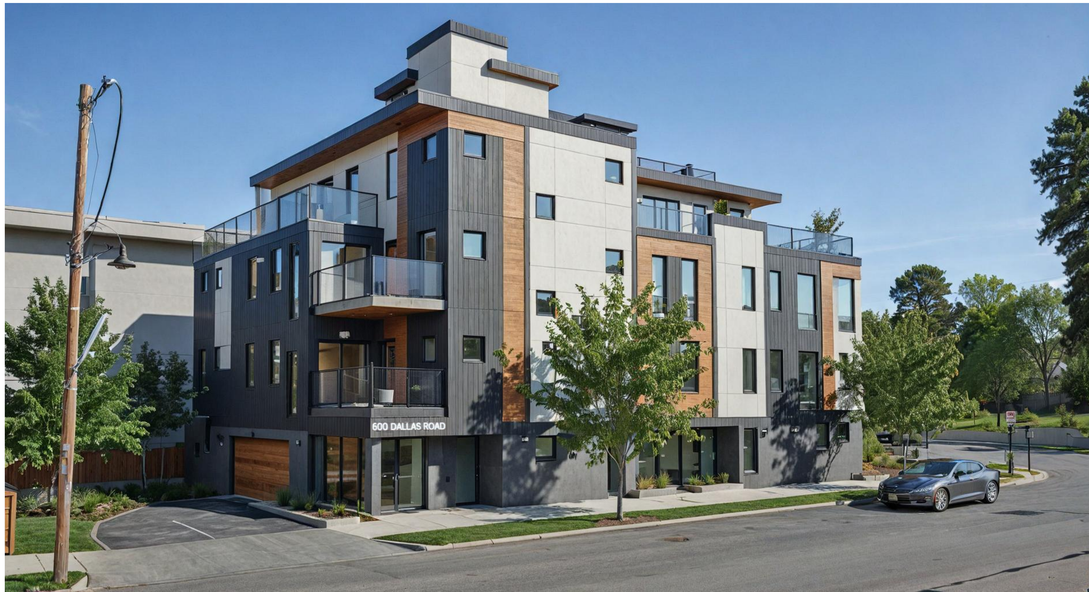
VIEW OF PROJECT FROM GOVERNMENT STREET
