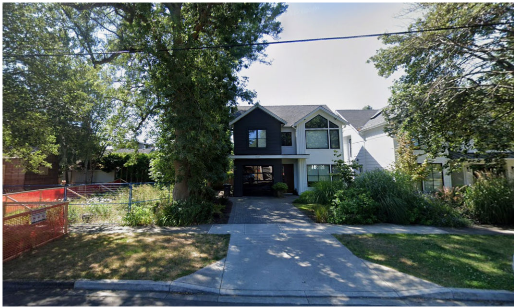
EXISTING STREET FRONTAGE: NEIGHBOURING PROPERTY ON CLIFFORD
