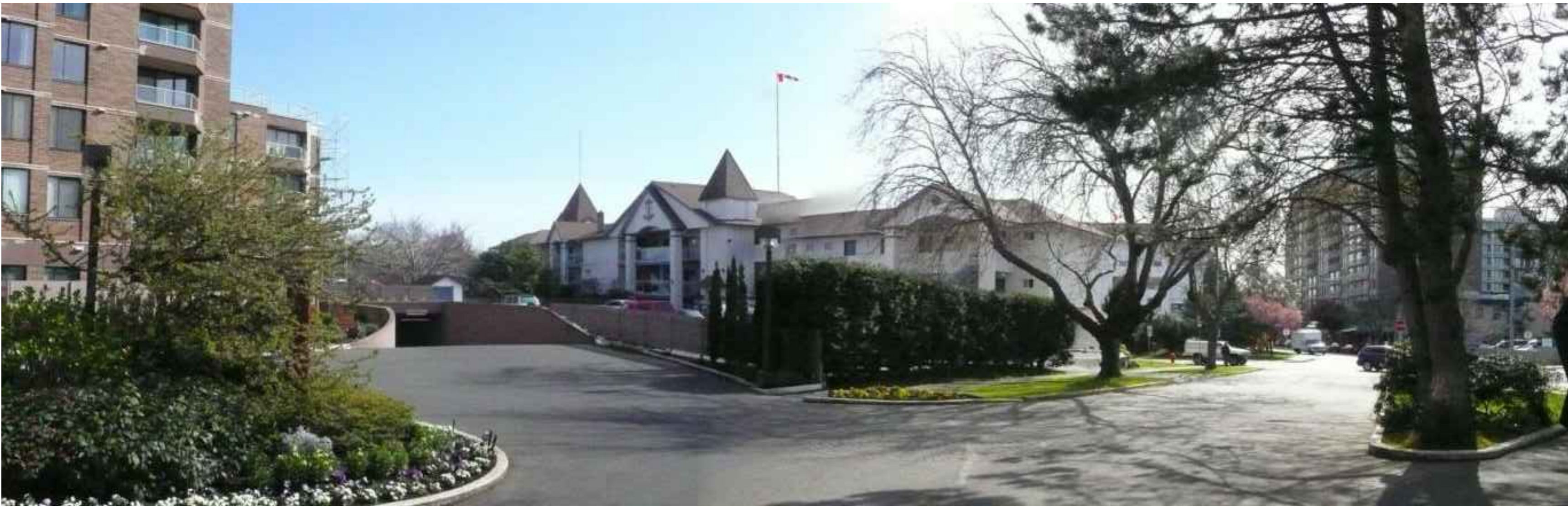
3 VIEW LOOKING SOUTH DOWN CROSS STREET NTS
