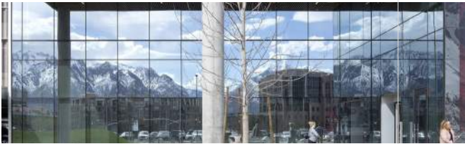
2 High Reflectance Glass High Performance Capped Curtain Wall
