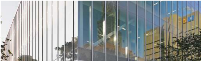
3 Low Reflectance Glass High Performance Capless Curtain Wall
