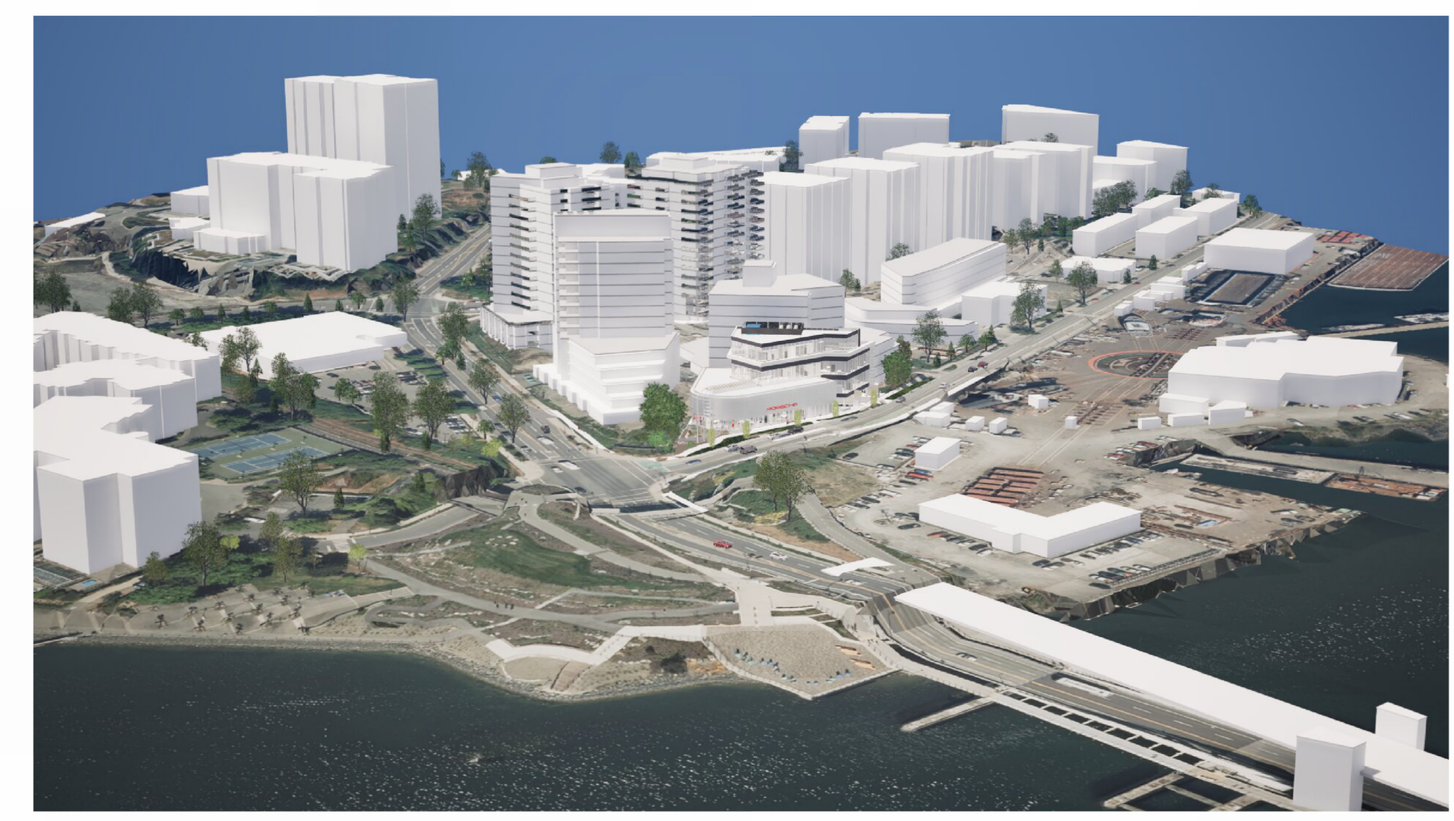
AERIAL VIEW FROM INTERSECTION OF ESQUIMALT ROAD AND HARBOUR ROAD
