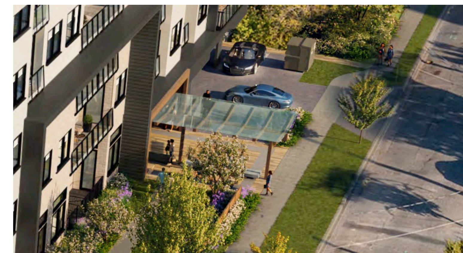
Main Entrance Plaza and Canopy
