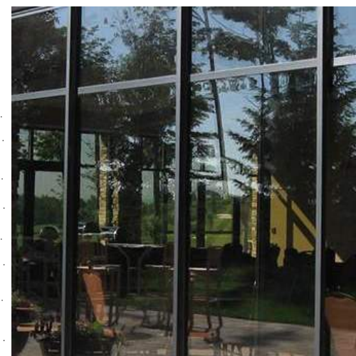
CW CURTAIN WALL BLACK MULLIONS
