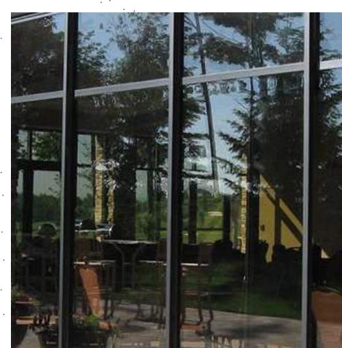
CW CURTAIN WALL BLACK MULLIONS
